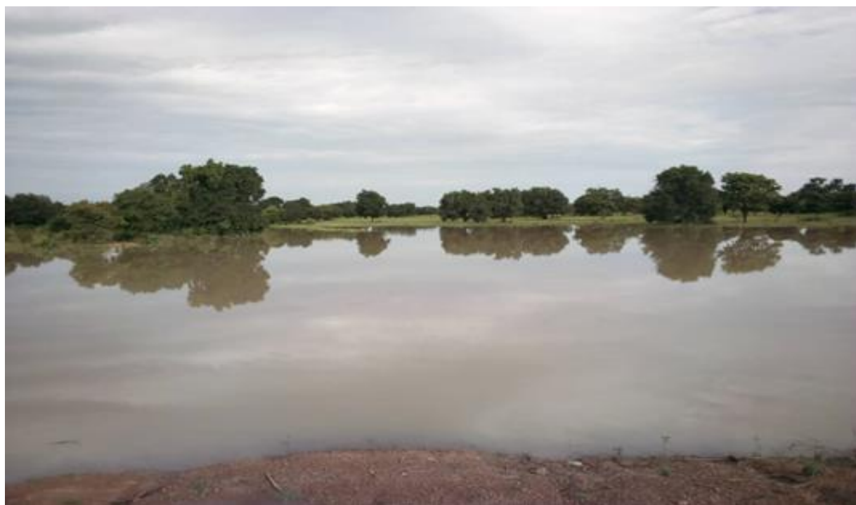
Fig 1.3 Rehabilitated 1No.Dug out
