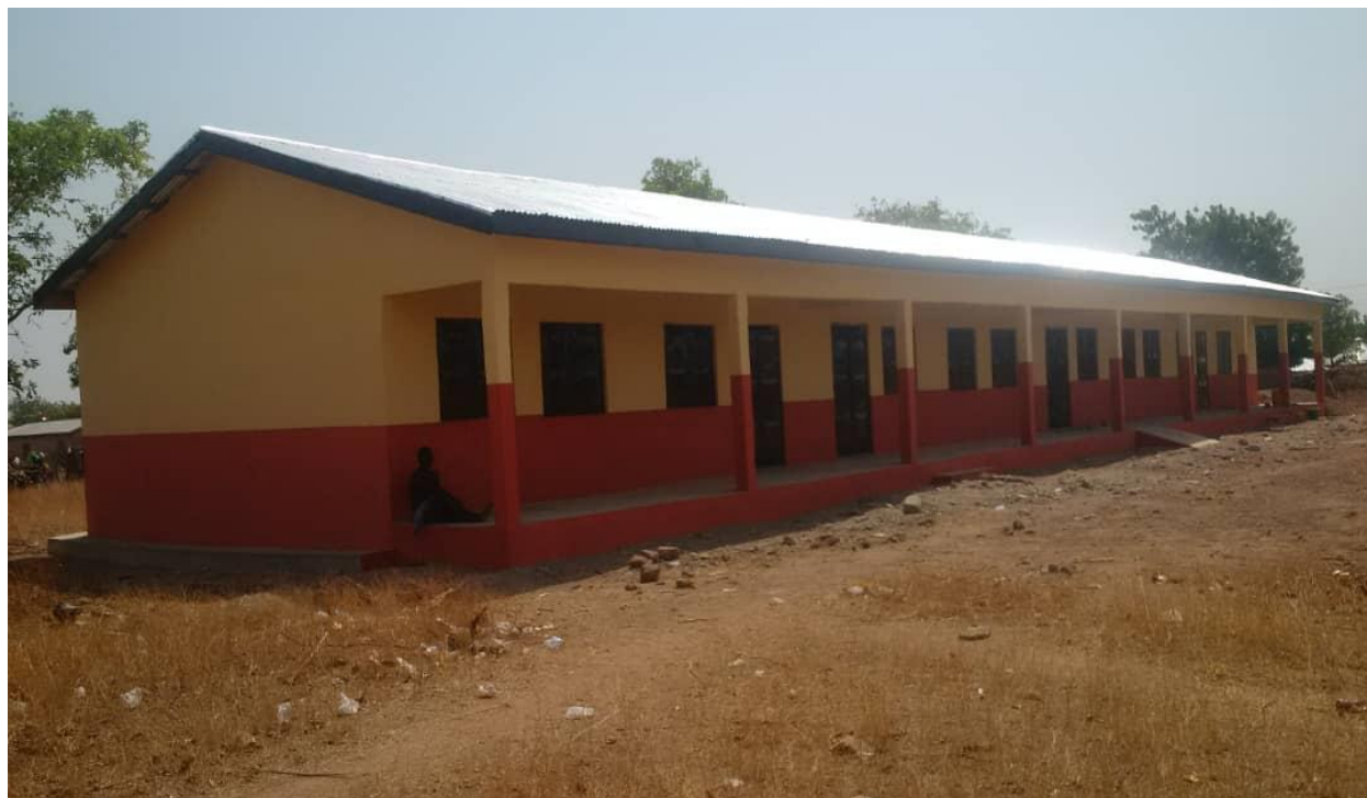
Fig. 1.1 Constructed 1No. 3-unit classroom block at Nabengu
