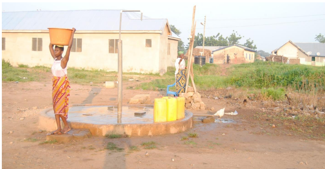
Fig. 1.5 Small Water System constructed at Sinsina and Kagbal
