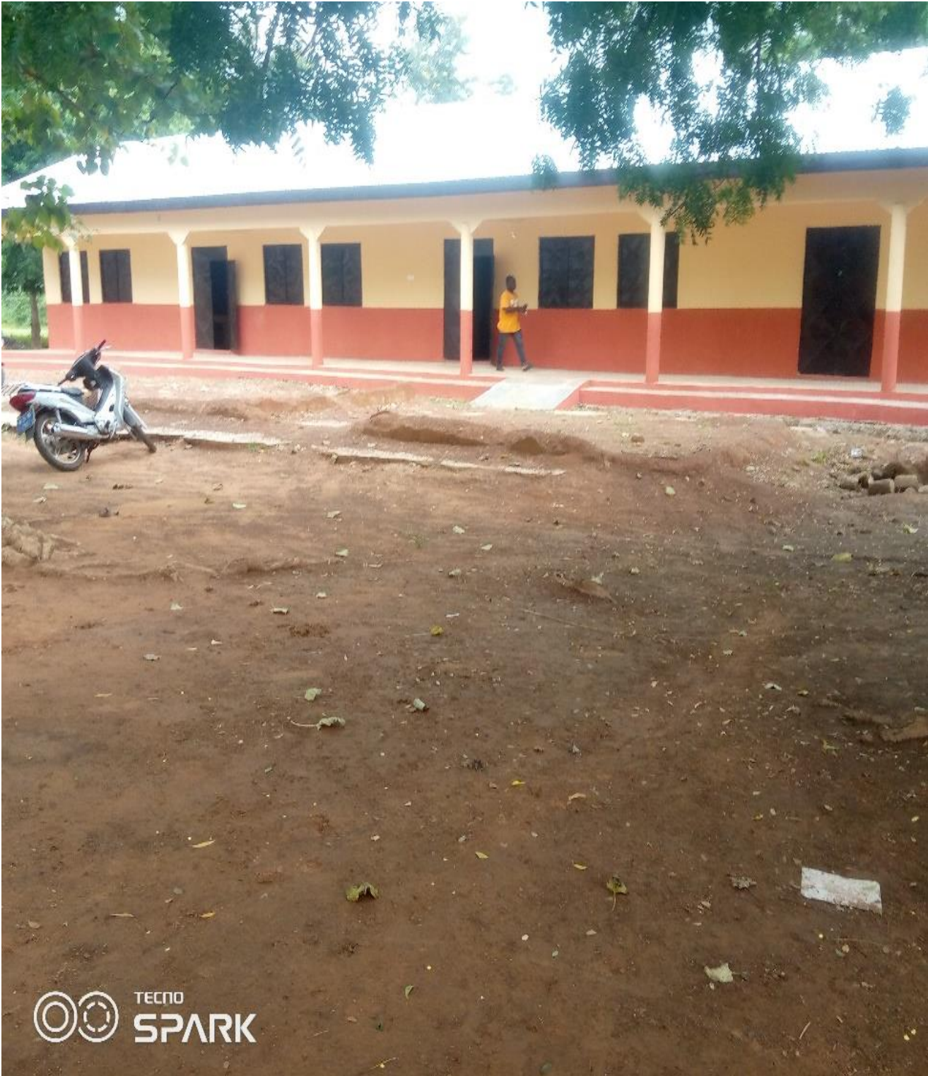
Newly Construted 3 no. Cl.asroom block at Zohe Community
