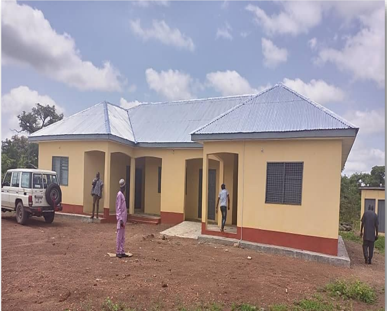
Figure 1: Constructed 1 No. CHPs Compound a
