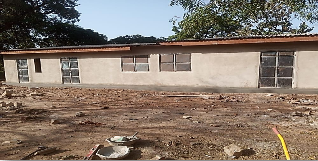
Figure 6: Ongoing Rehabilitation of 1 No. 3-Unit Classroom Block at Dakpam
