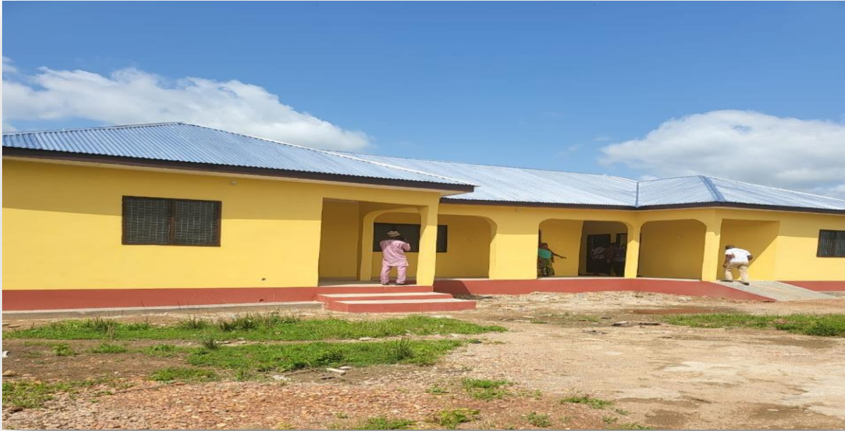
Figure 2: Constructed 1 No. CHPs Compound at Kanjonayili
