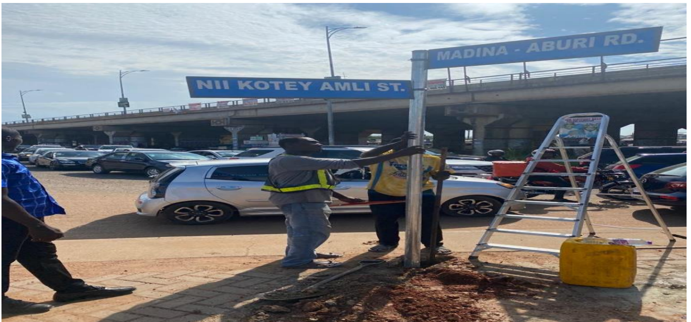
Figure 3: Installation of Street Signages at Atomic Junction
