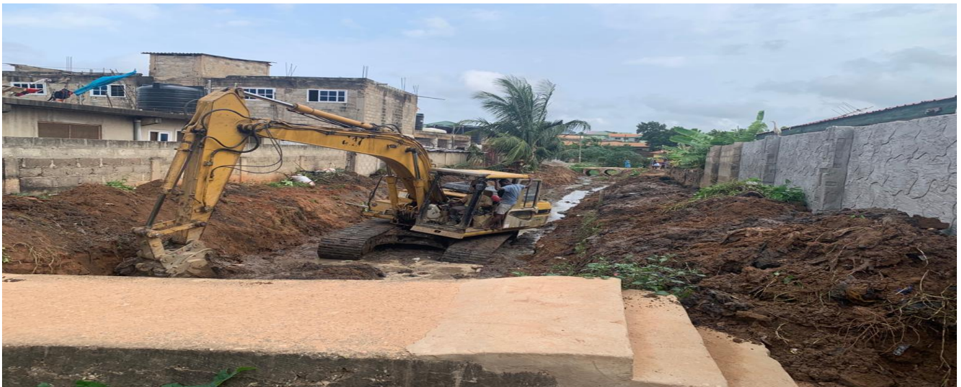
Figure 6: Dredging of 1.5km length of drains at Redco Down
