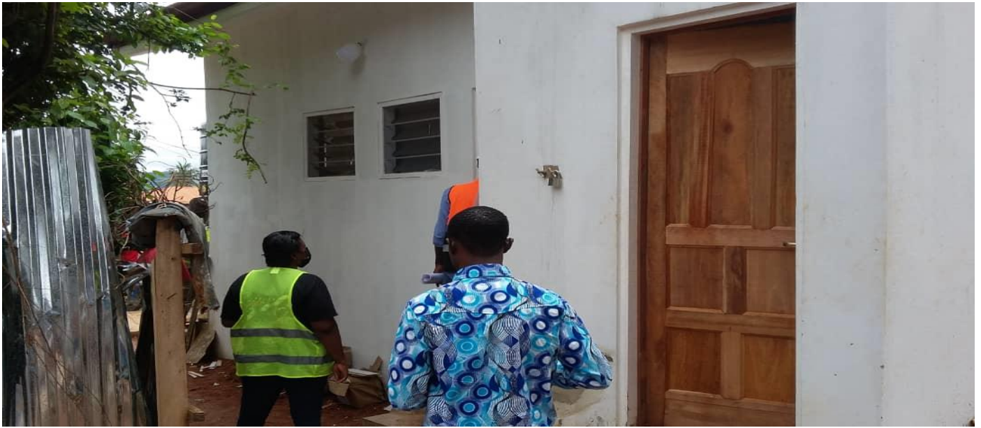
Figure 2: 12-Unit Improved Water Closet Institutional Toilet at Pantang Hospital
