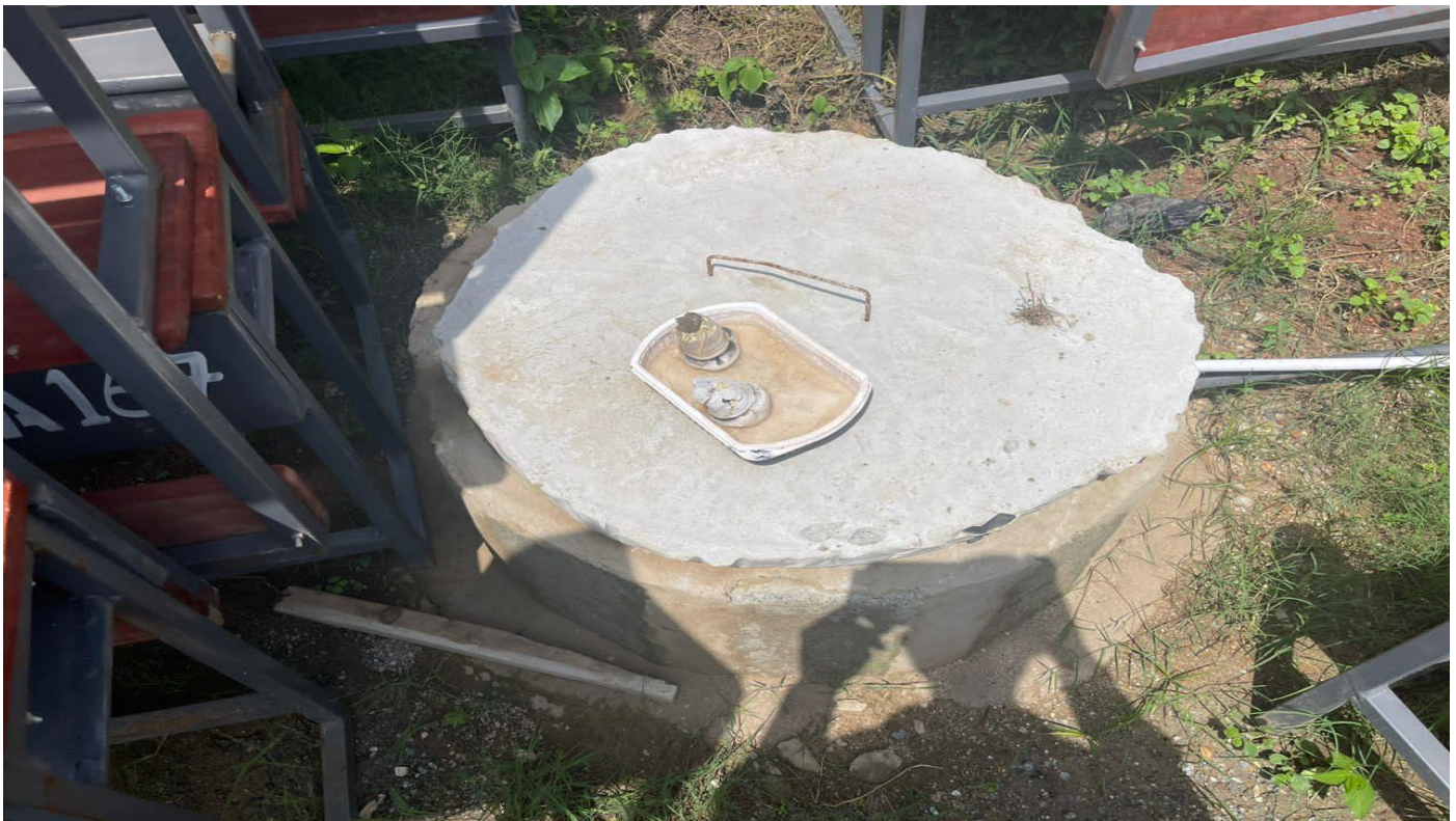
Figure 7: Mechanised Borehole at Madina Social Welfare
