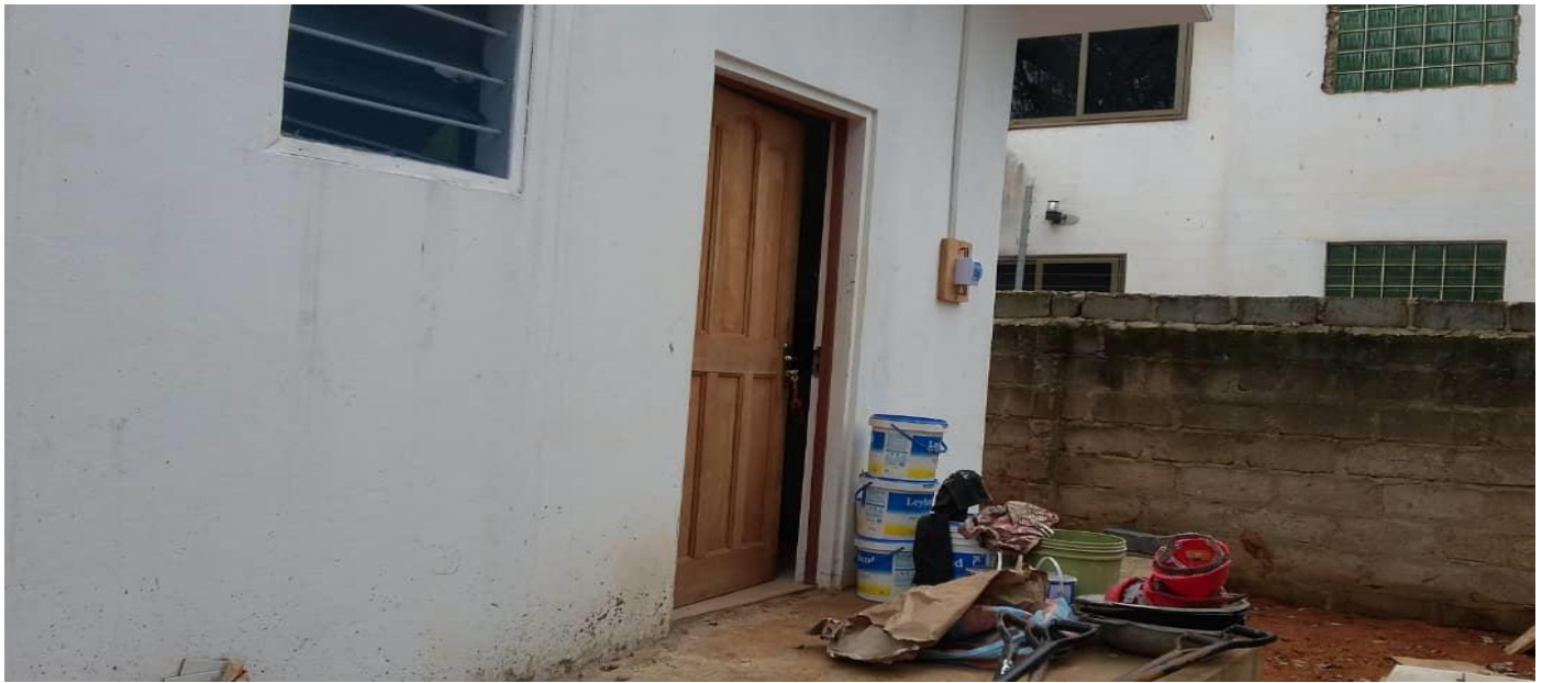
Figure 4: 5-Unit Improved Water Closet Toilet at Danfa Health Centre
