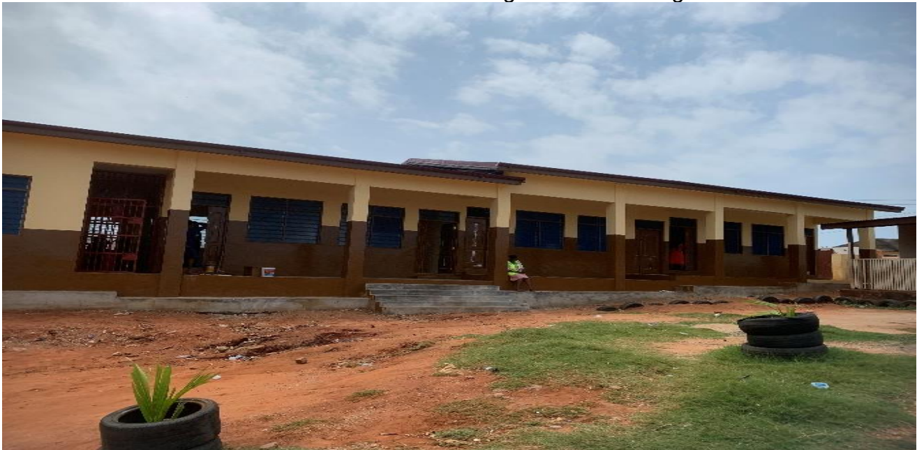
Completed 1 No. 3-Unit Classroom Block with Head teacher's Office, Storeroom and Staff Common Room at Nungua St Peters Anglican School
