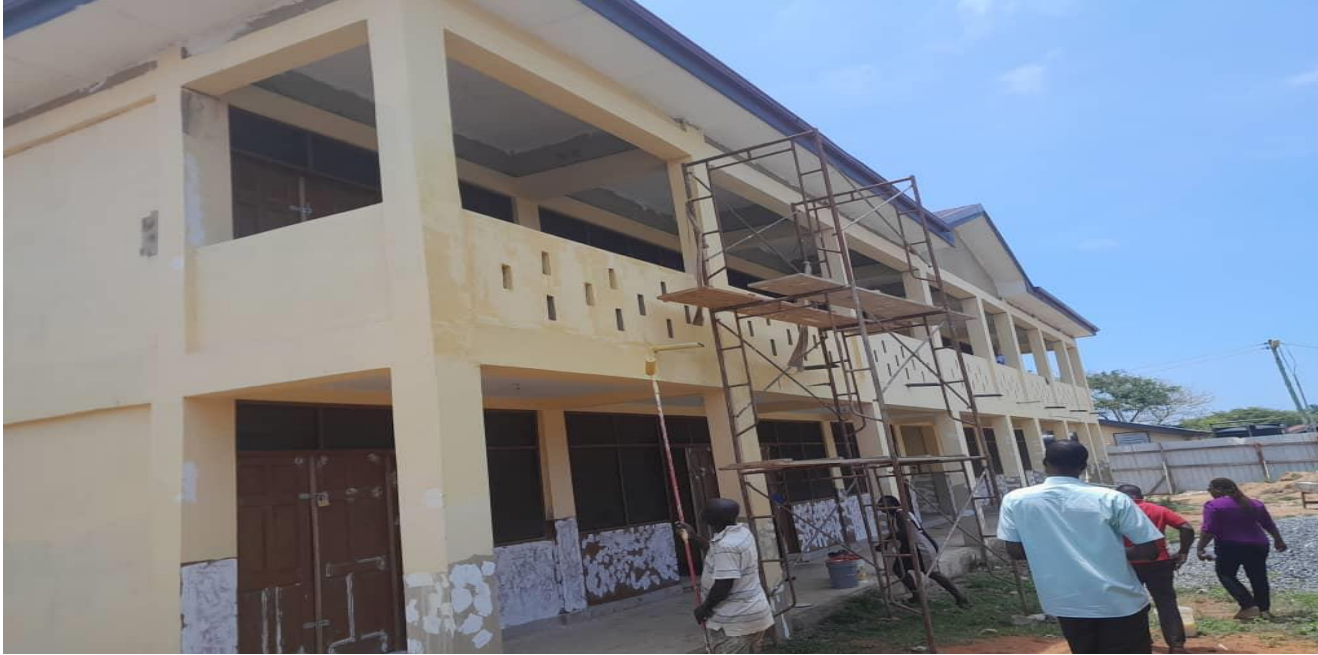
90% Completion of 2-storey 6-Unit classroom Block at Nungua Cluster of Schools
