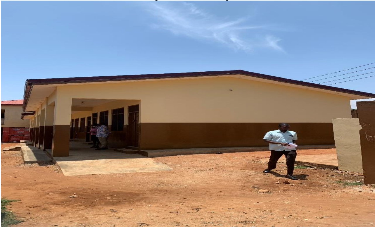
Completed 1 No. 3-Unit Classroom Block with Head teacher's Office, Storeroom and Staff Common Room at Nungua St Peters Anglican School
