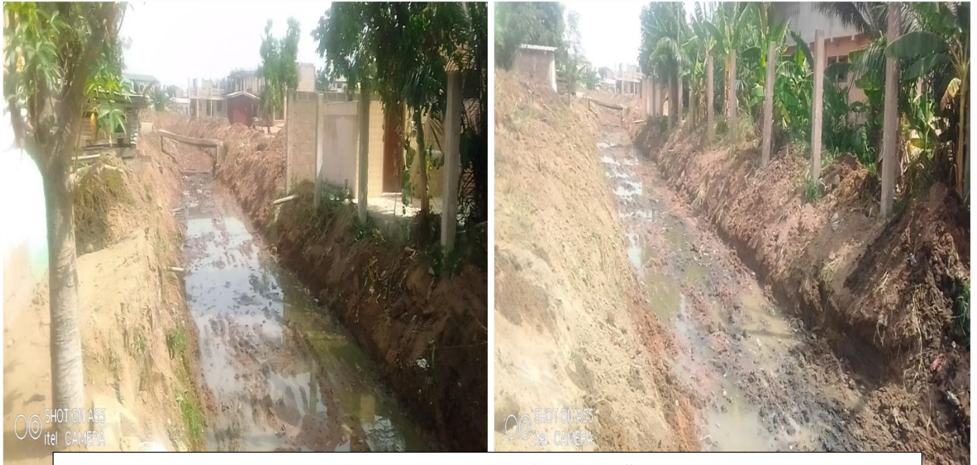
AFTER DREDGING WORKS
