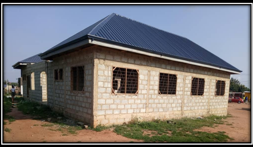
Construction of CHPS Compound at Domeabra
