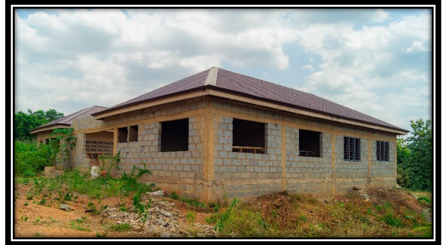
Construction of CHPS Compound at Fakyeneko
