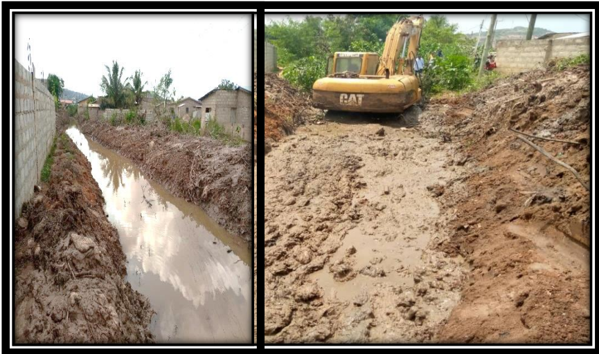
Dredging at Tuba and Amanfro
