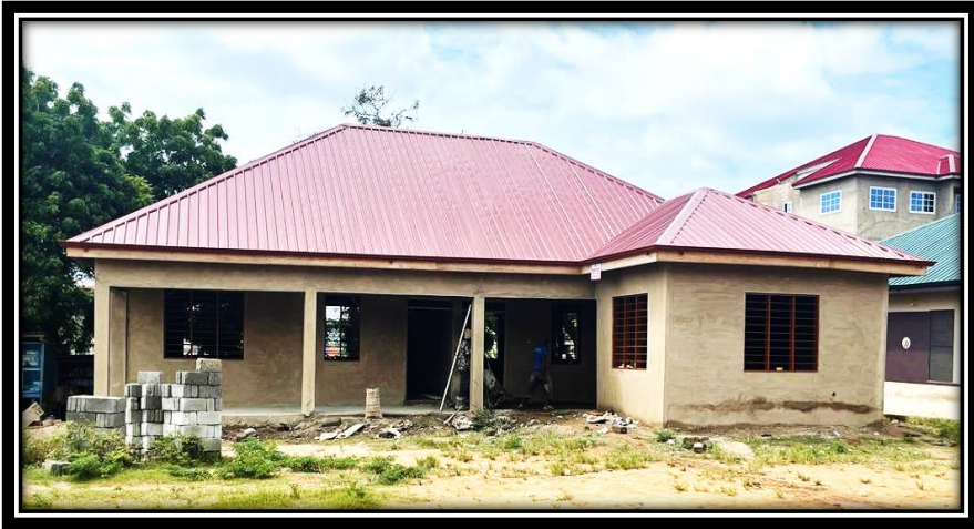
Const. of 1 No. 2 Unit Classroom Block at Bortianor
