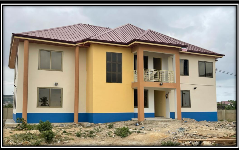
Construction of Police Divisional Headquarters at Tuba
