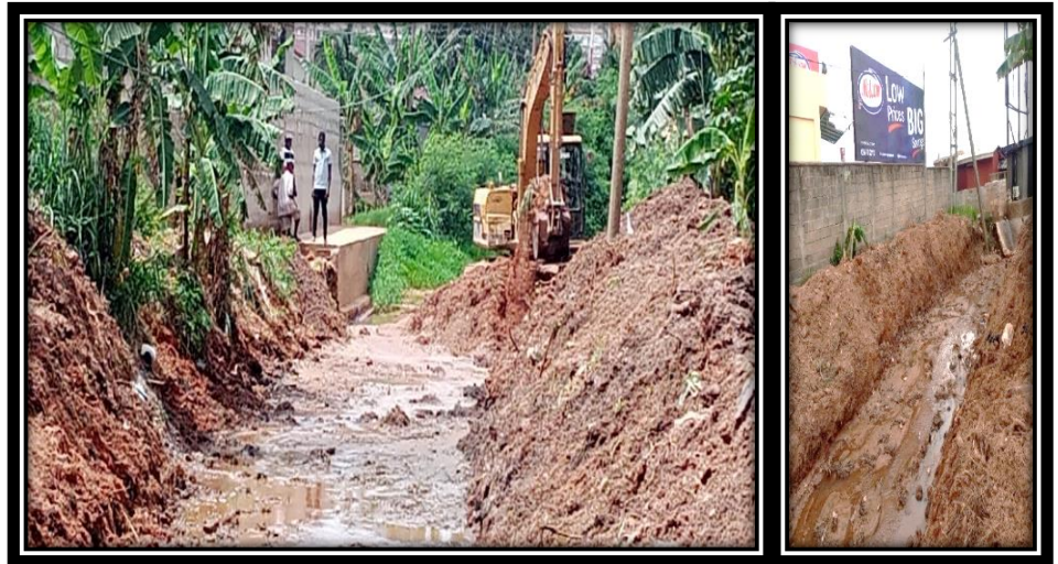
Dredging at Melcom
