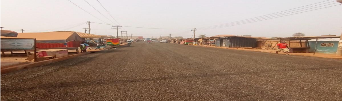
Constructed five no. roads
