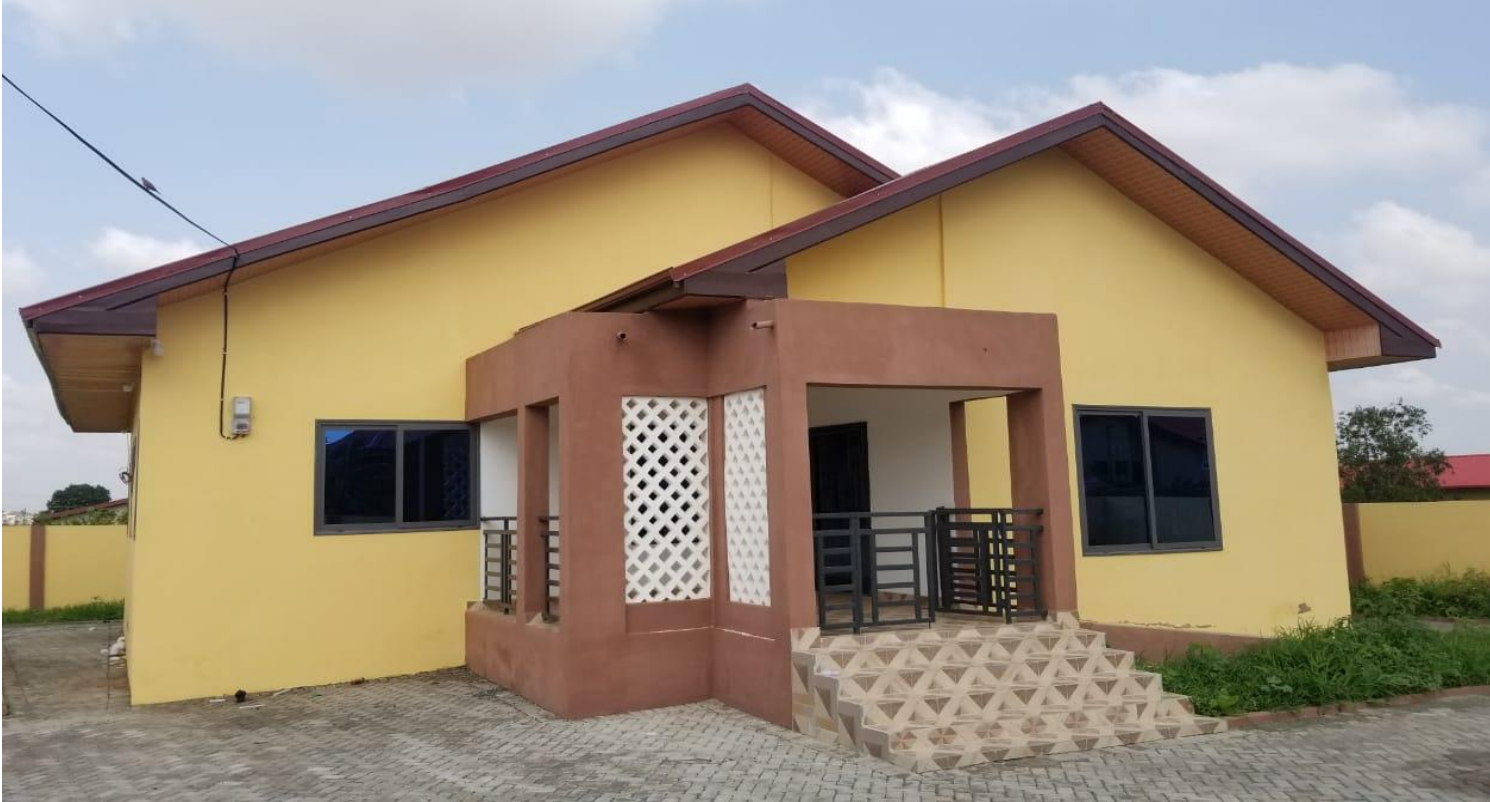
Constructed Bungalow for GES Director
