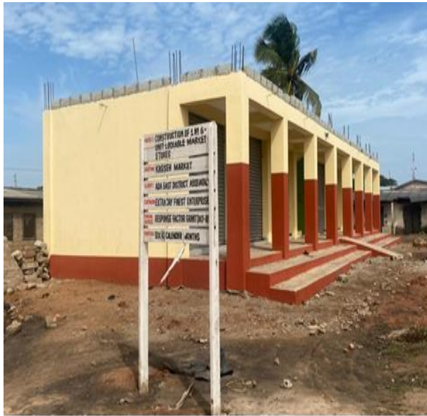
CONSTRUCTION OF 6-UNIT LOCKABLE MARKET STORES AT KASSEH MARKET
