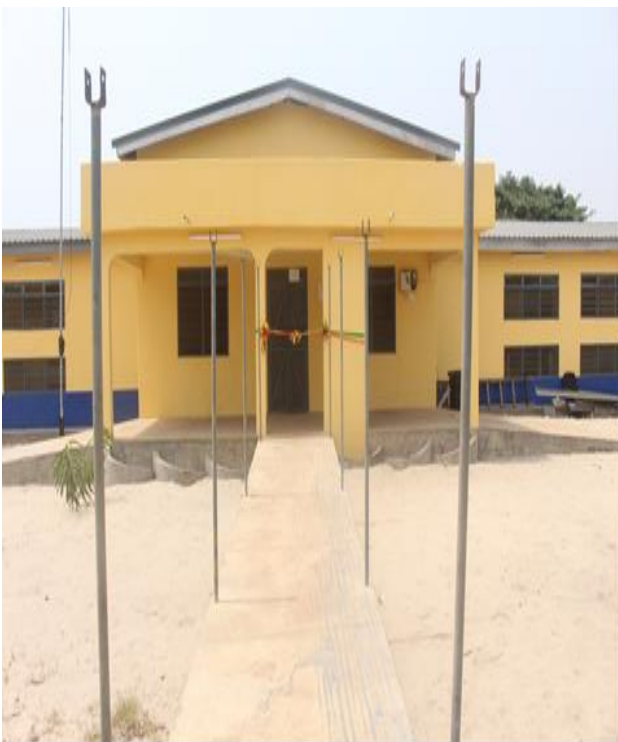
REHABILITATION OF RECOVERY WARD @ ADA FOAH HEALTH CENTER
