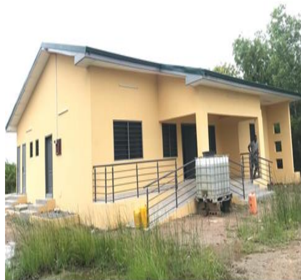
CONSTRUCTED 1NO. CHPS COMPOUND @ ALORKPEM
