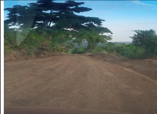
Reshaped 21km feeder road at Abisu No. 1, Tokrom and Sedan
