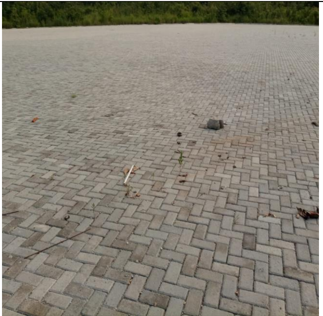
Completed 1No. Durbar Ground at Abene
