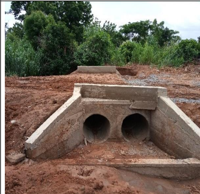
Constructed 3no. 900mm Culverts at Nkwakwasem
