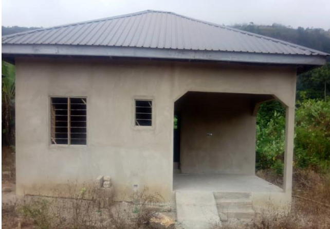
Completion 1No. CHPS Compound with Out-House at Abisu (70% Completed)
