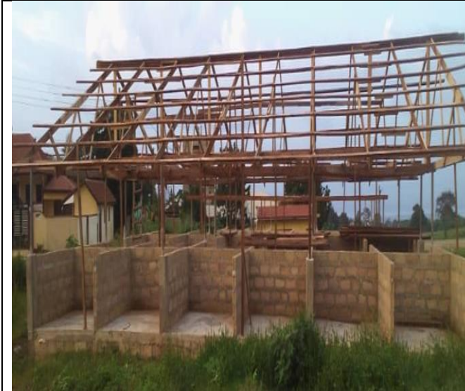
Completion of 2No. 24-Units Market Shed at Pepease. (70% Completed)
