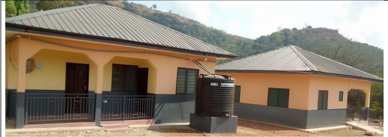
Completed 1No. CHPS Compound with Outhouse at Oframase.
