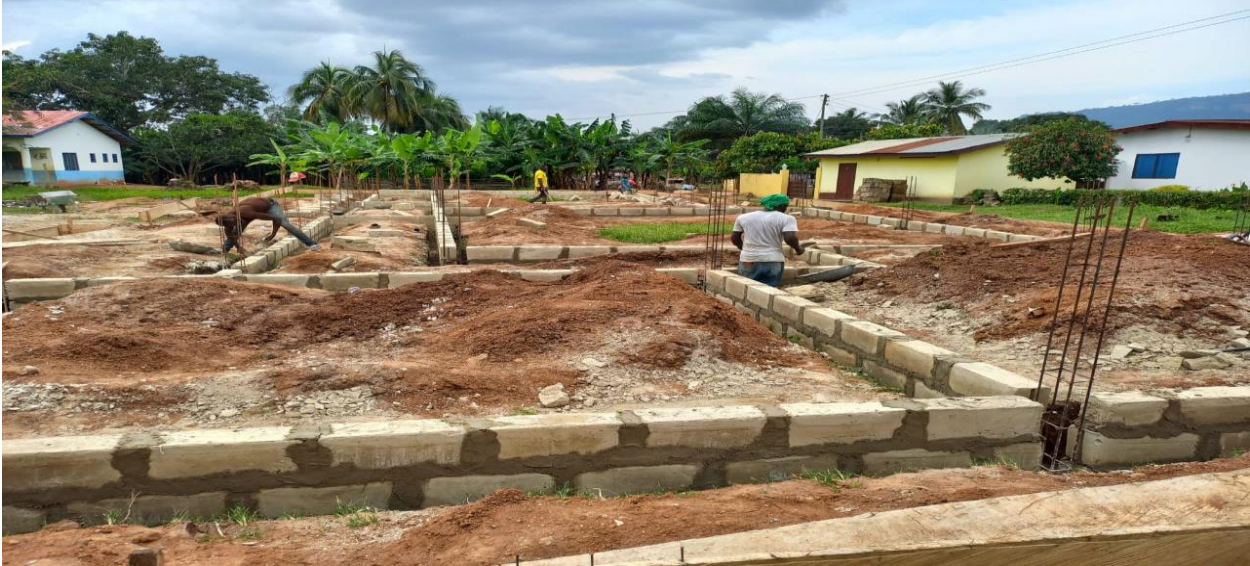
Hemang SDA JHS Block under construction
