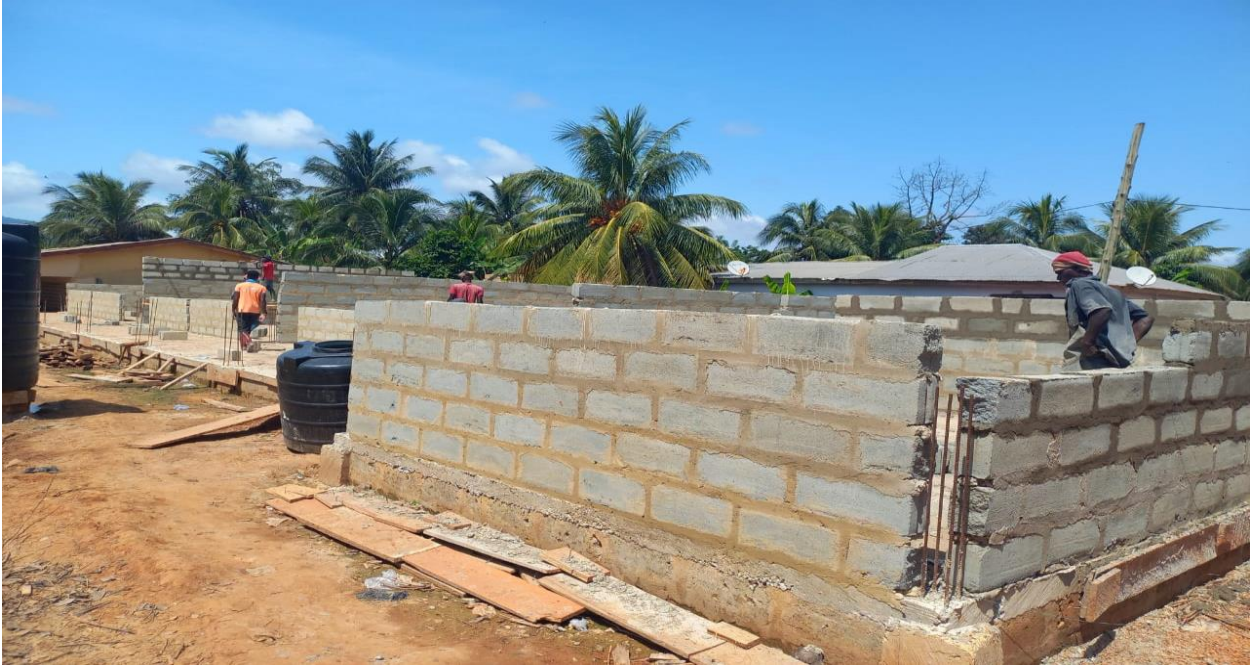
Nsutam SDA JHS Block under construction
