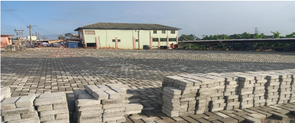
Construction floor pavement with kerbs and Sheds at Osino Lorry Park
