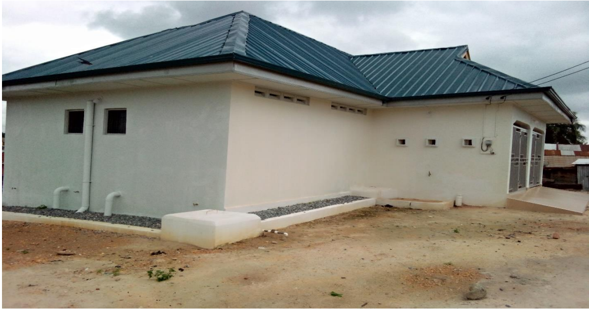
24-SEATER WATER CLOSET TOILET FACILITY FOR BOTH MALE AND FEMALE CONSTRUCTED AT AKIM ODA
