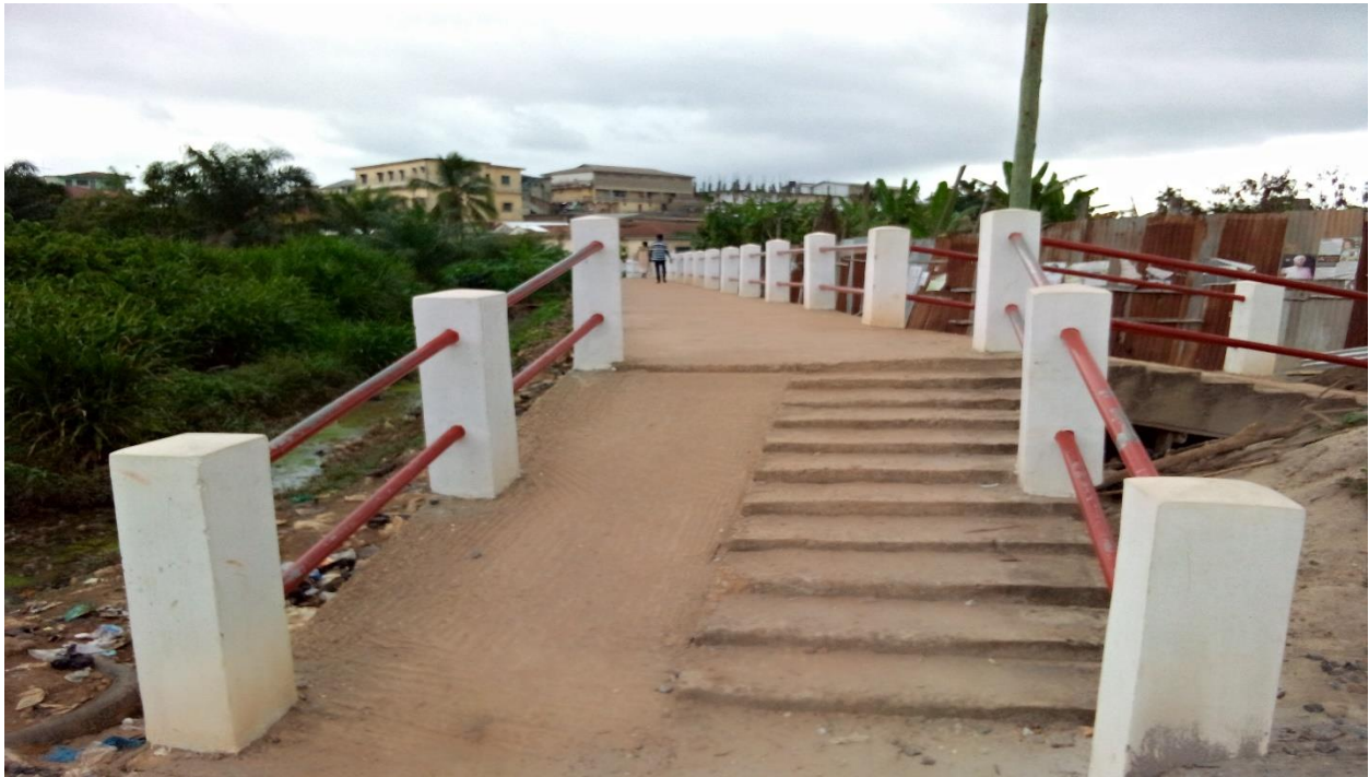
1NO. FOOT BRIDGE AT MADARINA, AKIM ODA CONSTRUCTED
