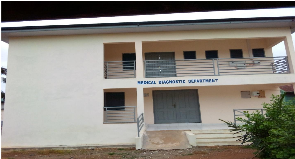
1NO. MEDICAL LABORATORY AT ODA GOVERNMENT HOSPITAL CONSTRUCTED
