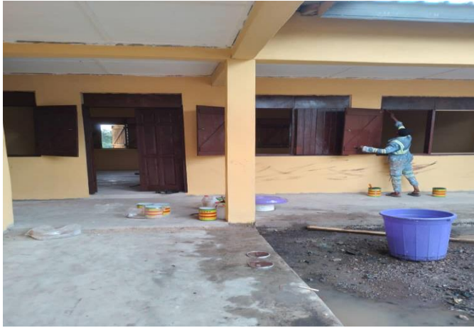
1No. 3unit classroom block at Ayensuadze (ASSEMBLY DACF)
