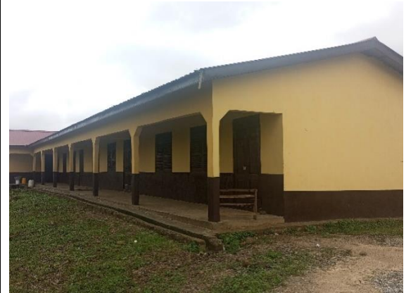
1No. 3unit classroom block at Oguaakrom (ASSEMBLY DACF)
