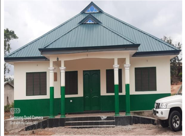
1No. CHPS compound at Mangoase (ASSEMBLY DACF)
