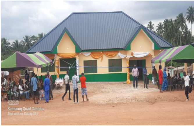
1No. CHPS Compound at Kwameadwer (ASSEMBLY-DACF)
