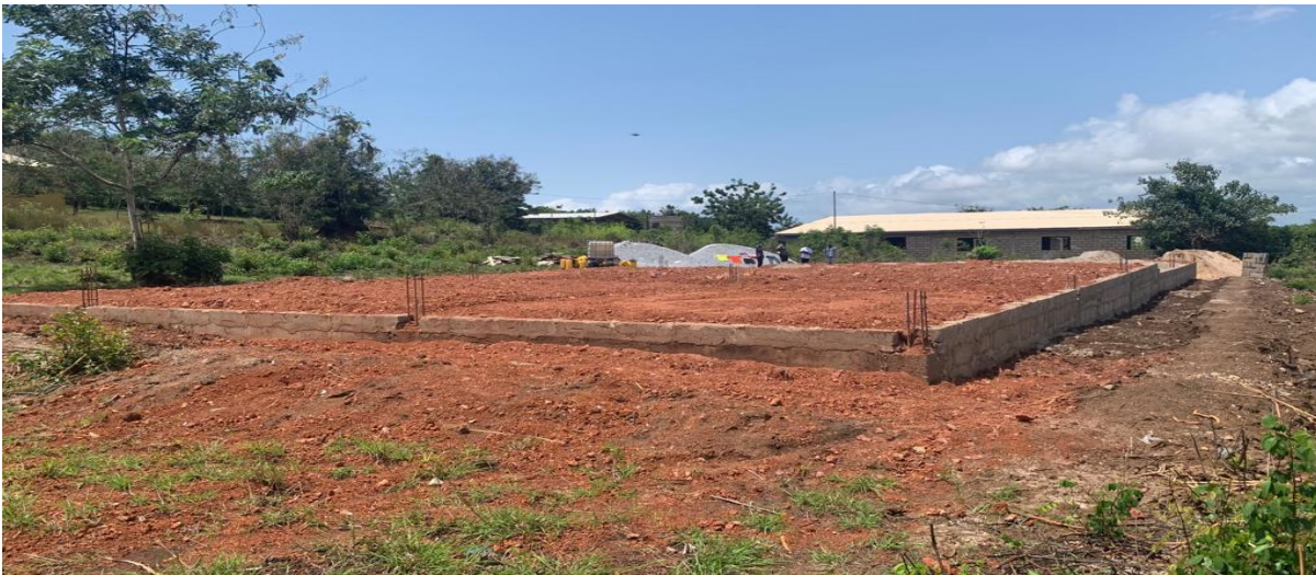
Figure 1: CONSTRUCTION OF 1 NO. 6-UNIT TEACHERS' QUARTERS AT GOMOA HWIDA
