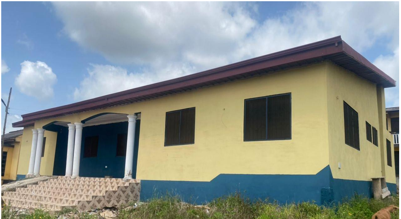
Completed Police Station in Berekum (Charge Office) – DACF-RFG
