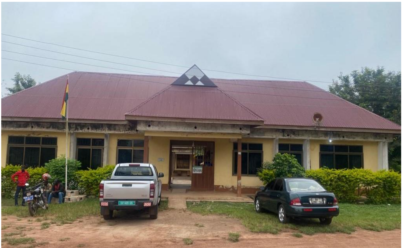
(Renovated GES office block) - - DACF
