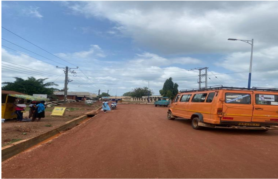
(Tarred 243m road, installed street lights, 1No. Traffic light and transformer at Berekum Thursday Market) - - GSCSP
