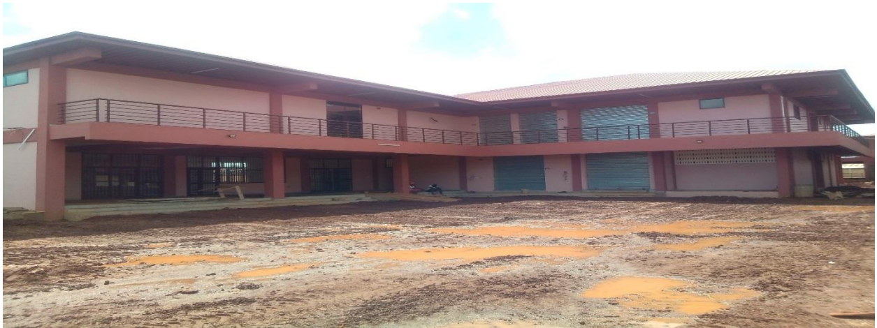
Completed 1no Market Store & Eatery (Block B) Nana Abena Market
