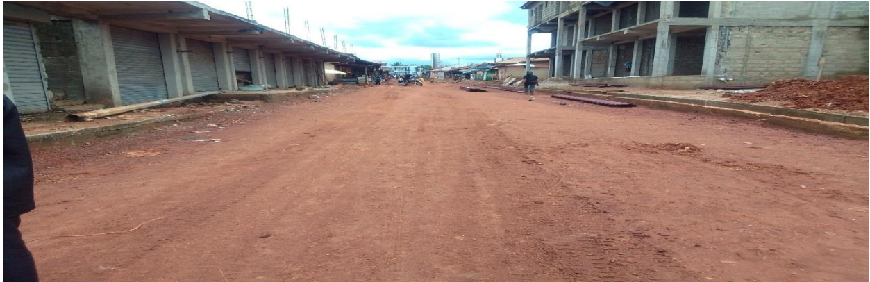
Constructed DVLA – Agyeiwaa road with 50% completion (UDG project)
