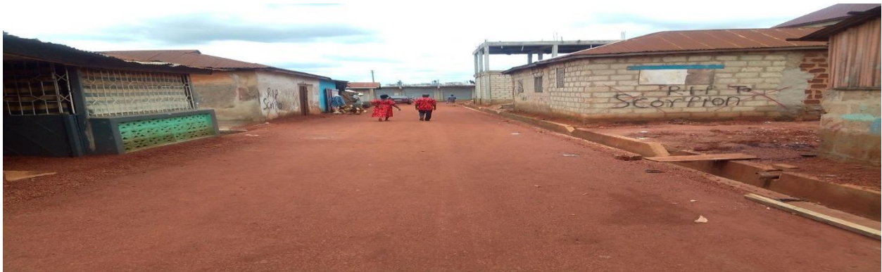
Constructed Techiman - Abanimu road with 50% completion (UDG project)
