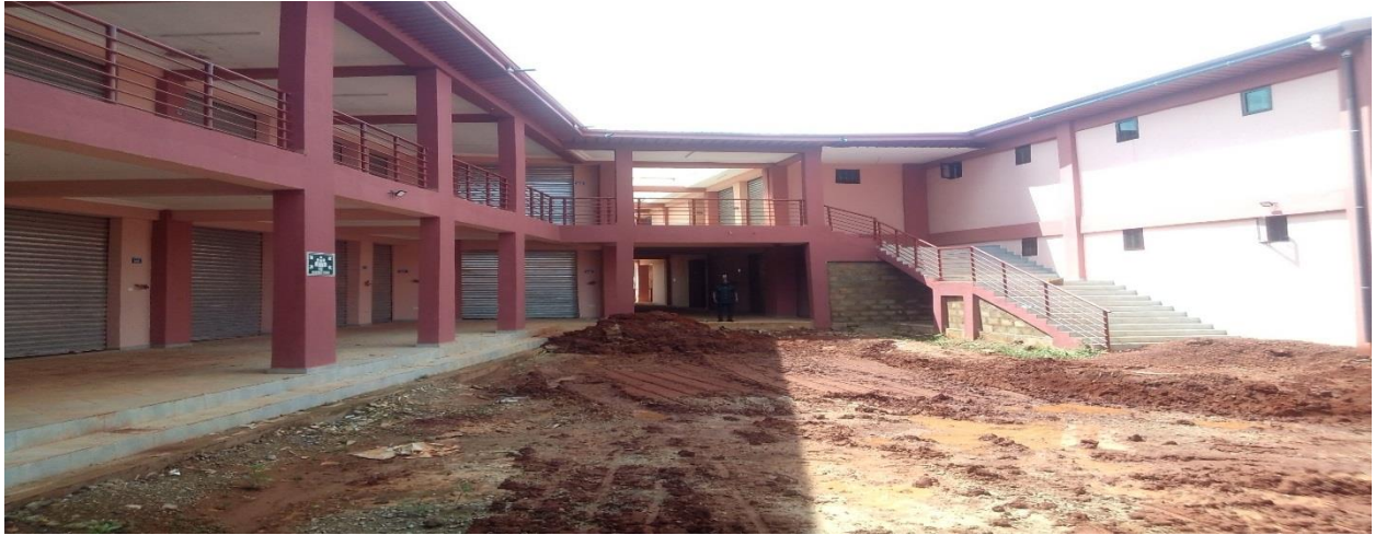
Completed 1no. Market Store Block A, at Nana Abena Market
