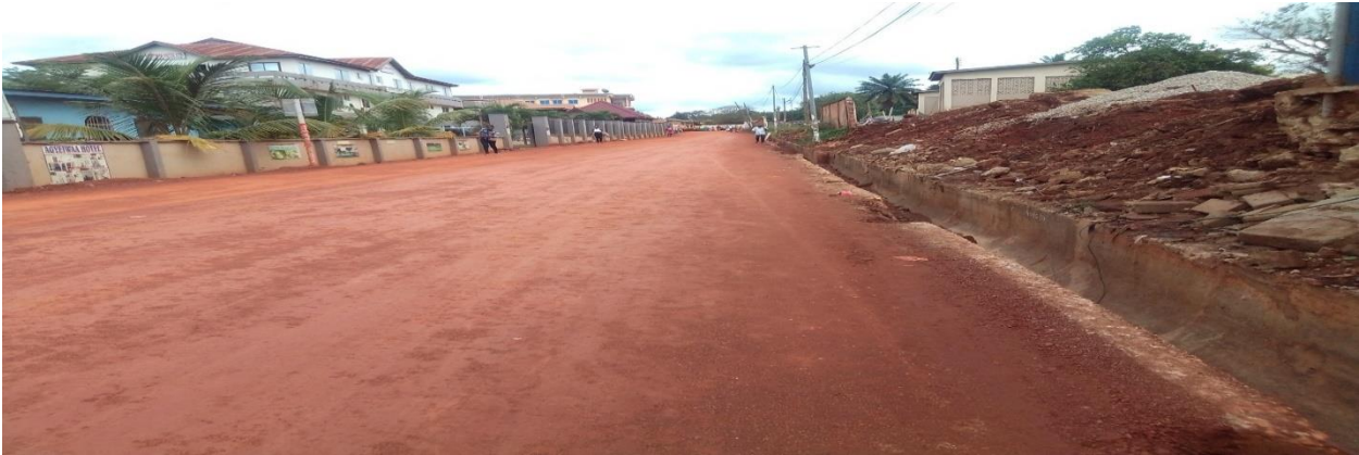
Constructed DVLA – Agyeiwaa road with 50% completion (UDG project)
