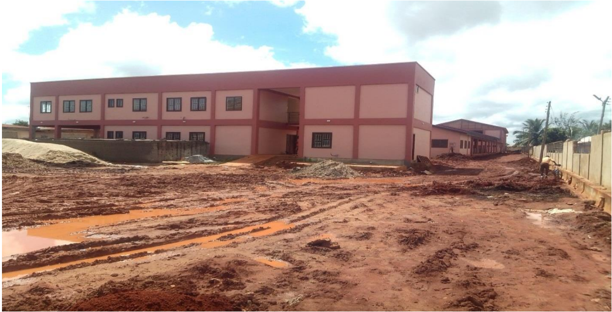
Completed 1no Administration Block (Block D) at Nana Abena Market
