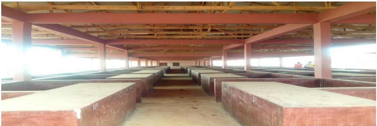
Completed 1no Market Sheds (Block C) at Nana Abena Market
