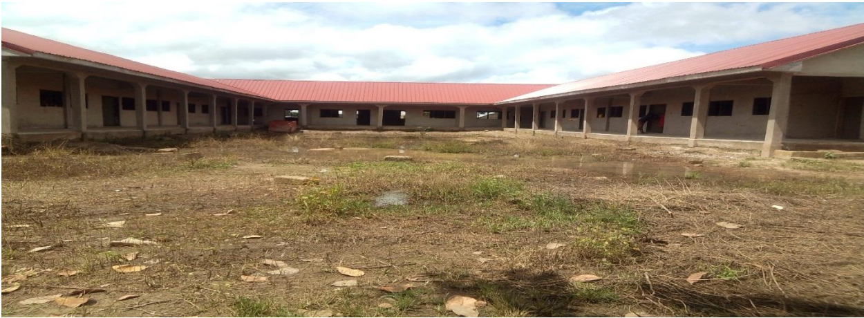
Constructed 1no 6-unit Classroom Block at New Jerusalem, Techiman – 70% completed
