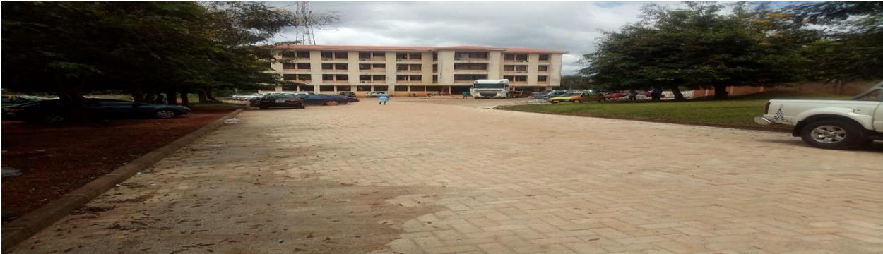
Paved Techiman Municipal Assembly forecourt, driveway, and drainage construction – 70% completed
