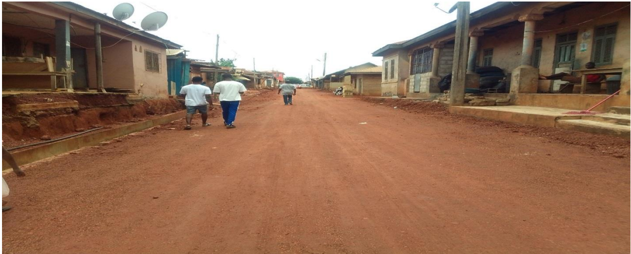
Constructed Techiman - Abanimu road with 50% completion (UDG project)
