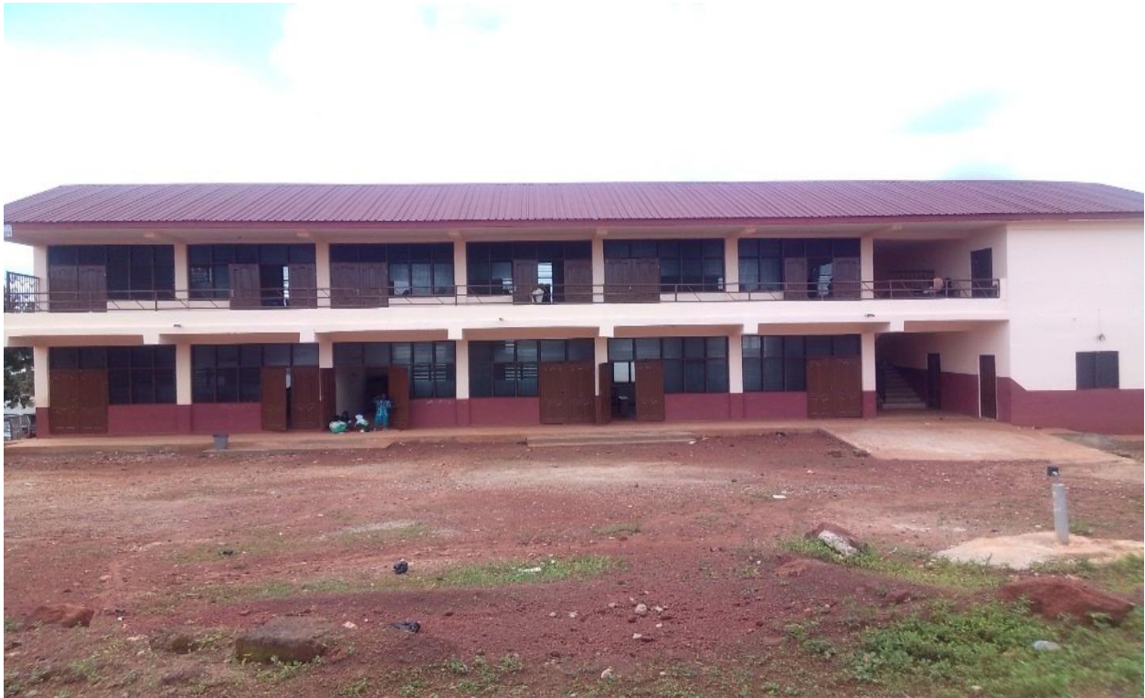
Completed 1no 6-unit Classroom Block at Kenten – Anyinabrem in Techiman
