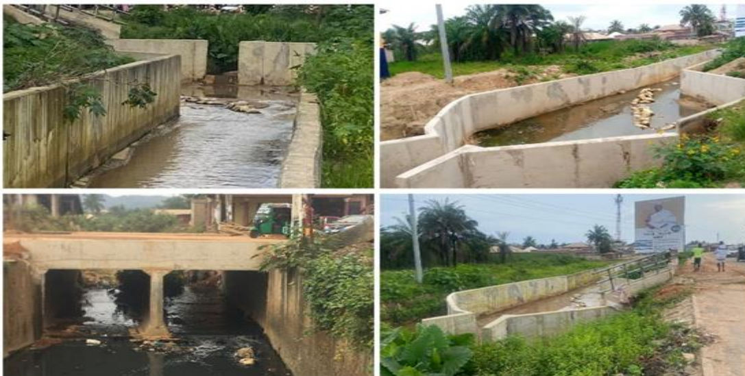
Construction of reinforced concrete 3.5 x 2m storm drains
