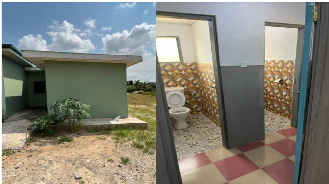
CONSTRUCTION OF TOILET FACILITY FOR SANSO HEALTH CENTRE
