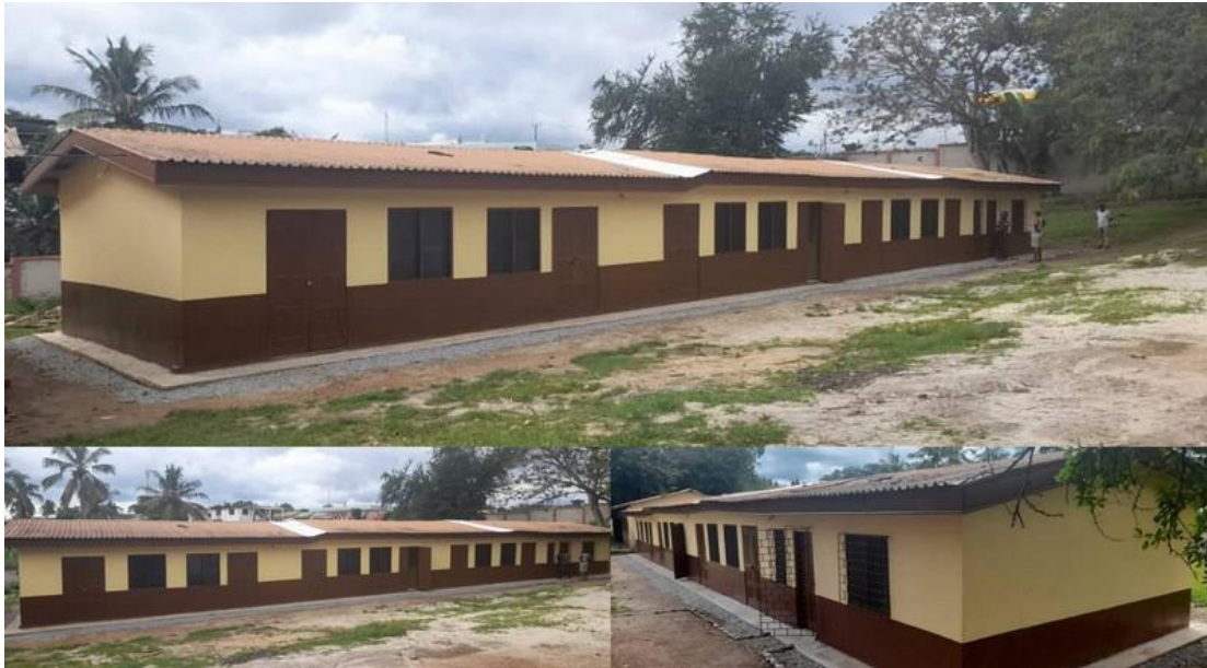
RENOVATED CLASSROOM BLOCK-NEW NSUTA
