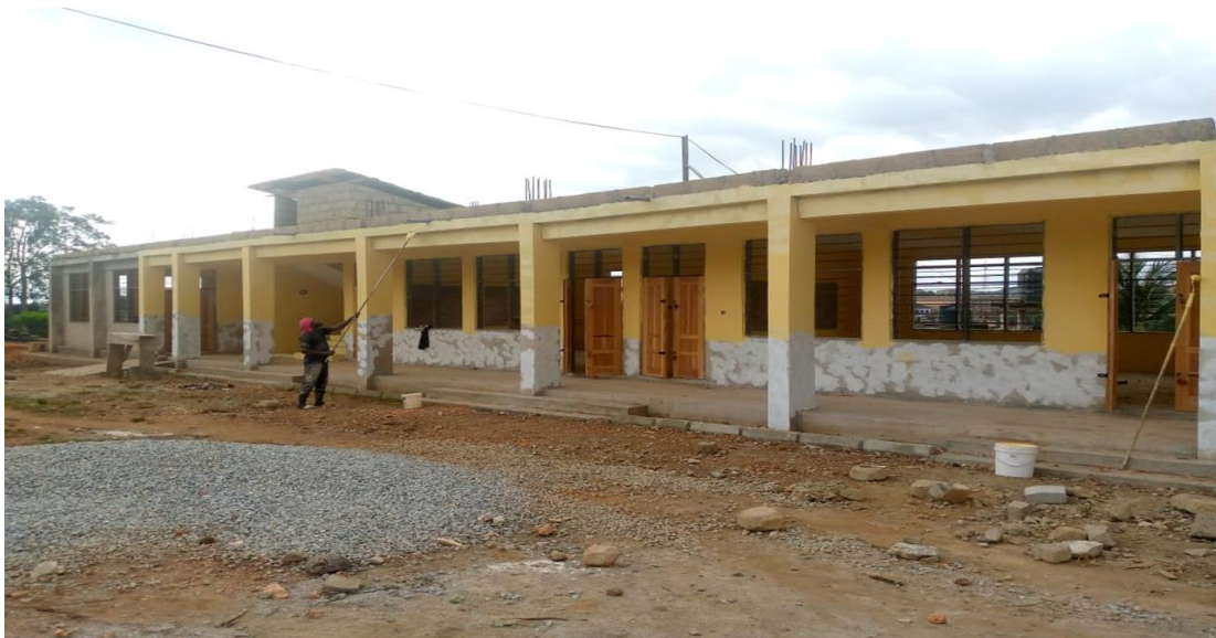
CONSTRUCTION GROUND FLOOR – 6 UNIT CLASSROOM BLOCK WITH ANCILARY FACILITIES AT BOGOBIRI
