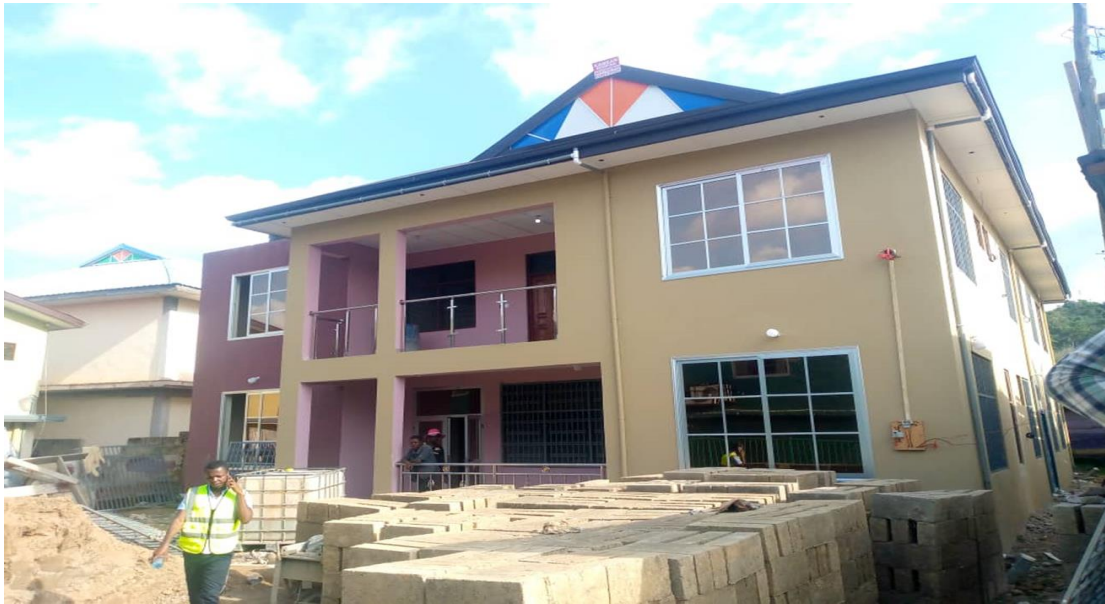
CONSTRUCTION OF CLINIC AT NEW NSUTA AUNTIE BEE
