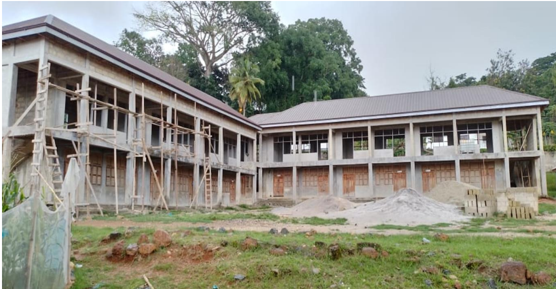
COMPLETION OF SECOND FLOOR 6 UNIT CLASSROOM BLOCK AT METHODIST SCHOOL (ANTOBOASI)
