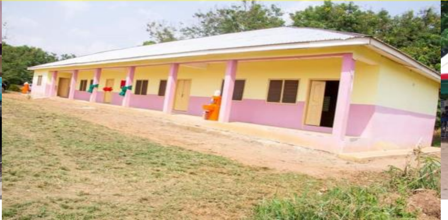
2NO. 2-UNIT KG BLOCK WITH STAFF OFFICE, STORE, W/C, CHANGING ROOMS SCHOOL AT NZIMA CONSTRUCTED AND FURNISHED (DACF)
