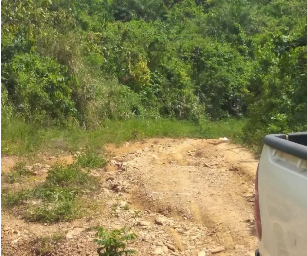
Reshaping of Yapesa to Adeito Feeder Road Before
