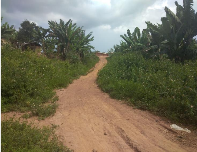
Reshaping Of Yapesa to Nkwantapong Feeder Road Before
