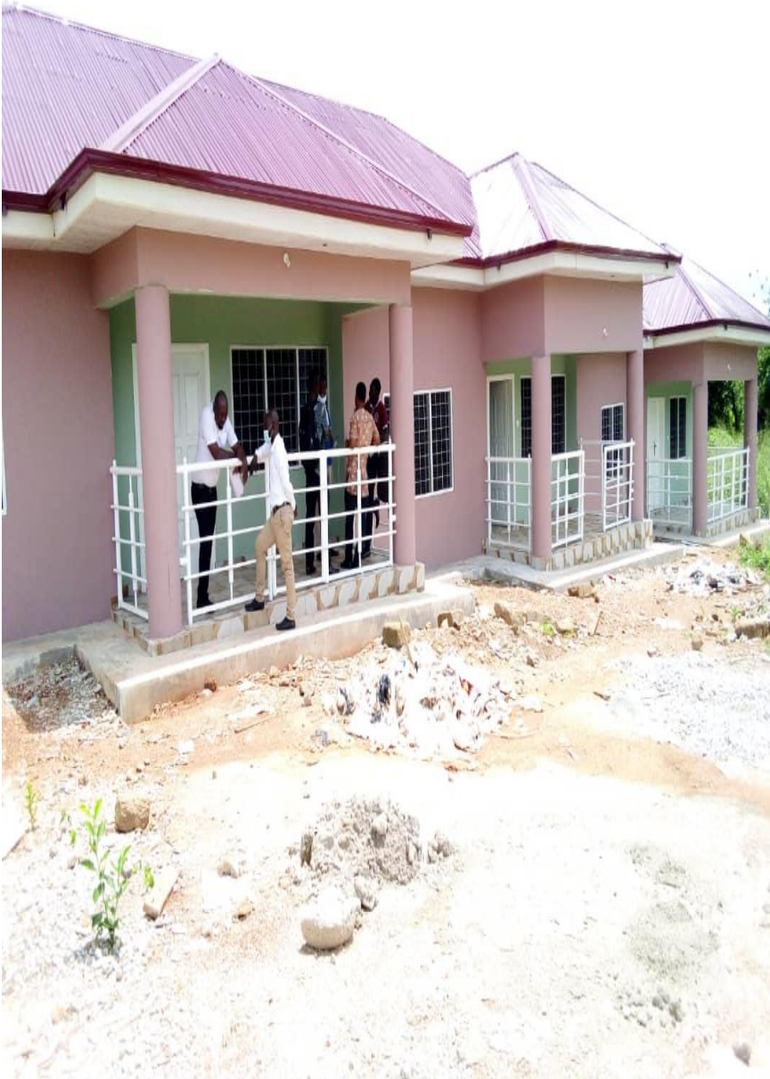
Constructed 3-Unit, One Bedroom with Hall, Kitchen, Toilet and Bath Nurse's Quarters. Adugyama Funded by DPAT
