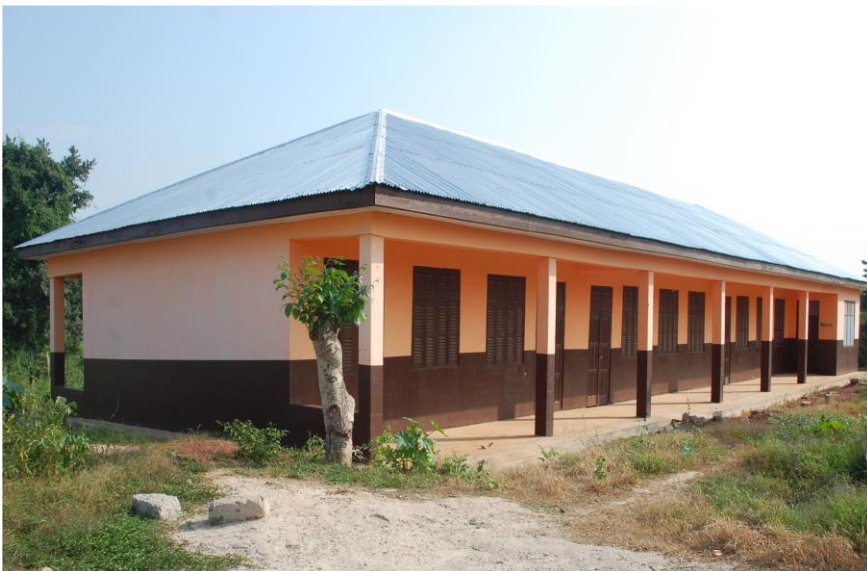
Constructed and Furnished 3-unit Classroom Block with Office, Store, Staff Common Room, 4-Seater KVIP and 2-Unit Urinal at Kwadokrom (Funded by: DACF)
