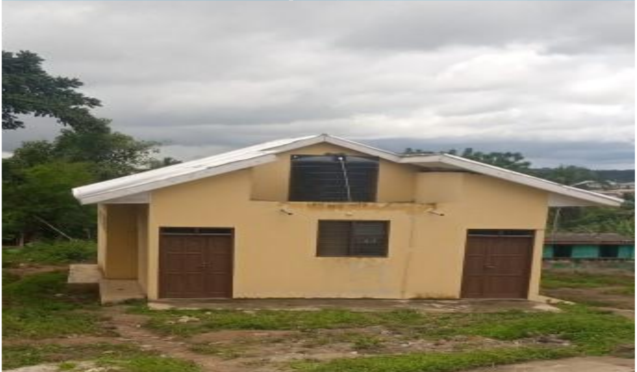
Constructed 1No. 16 seater WC Toilet with Mechanized Borehole . Dompoase (DACF)
