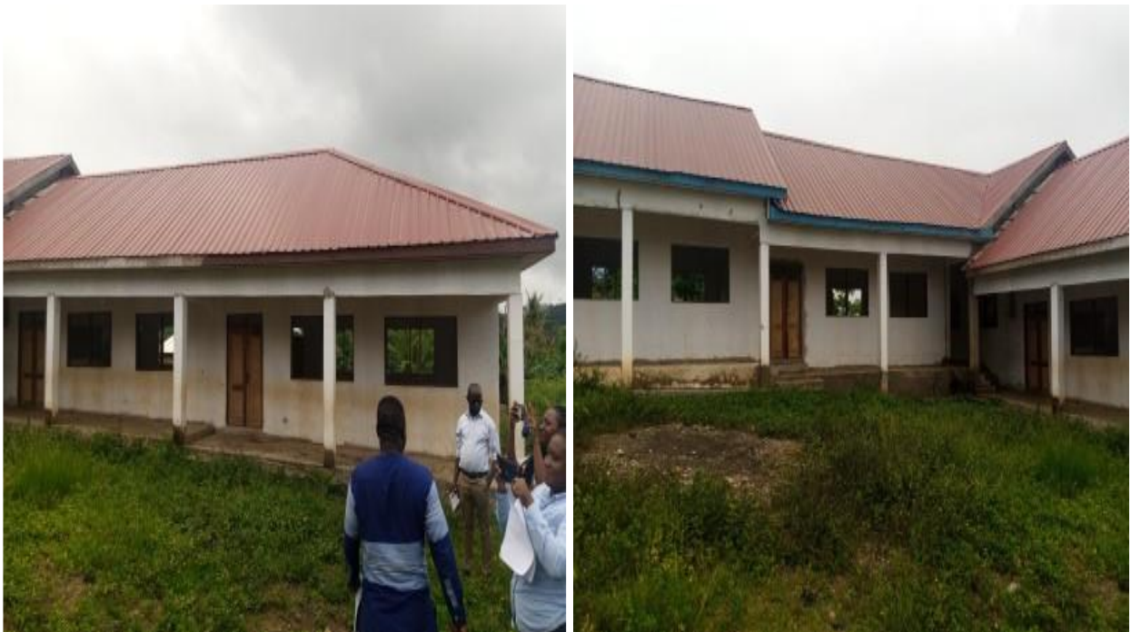
Constructed 1No.3 Unit Classroom Block with ancillary facilities. Adokwai (DACF)
