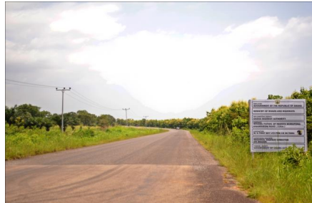
6. Ongoing construction of 12km road from Wurupong to Kwamekrom
