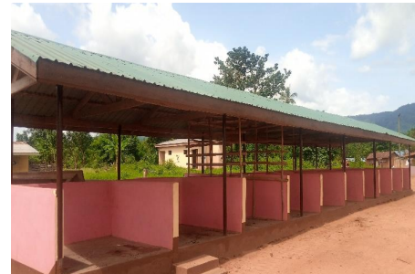
13. Completed a 20-unit market shed from IGF at Bumbula
