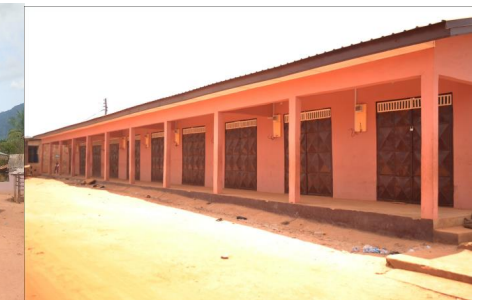
14. Ongoing construction of 20-unit lockable stores at Kwamekrom
