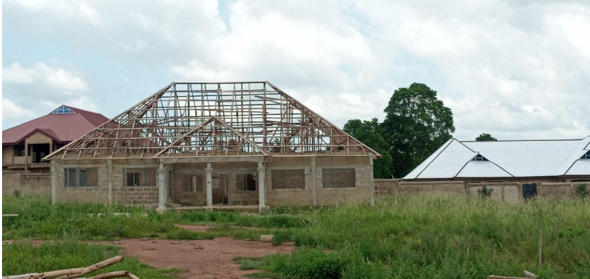
Figure 7: Construction of Dress Room at Wenchi Sports Field
