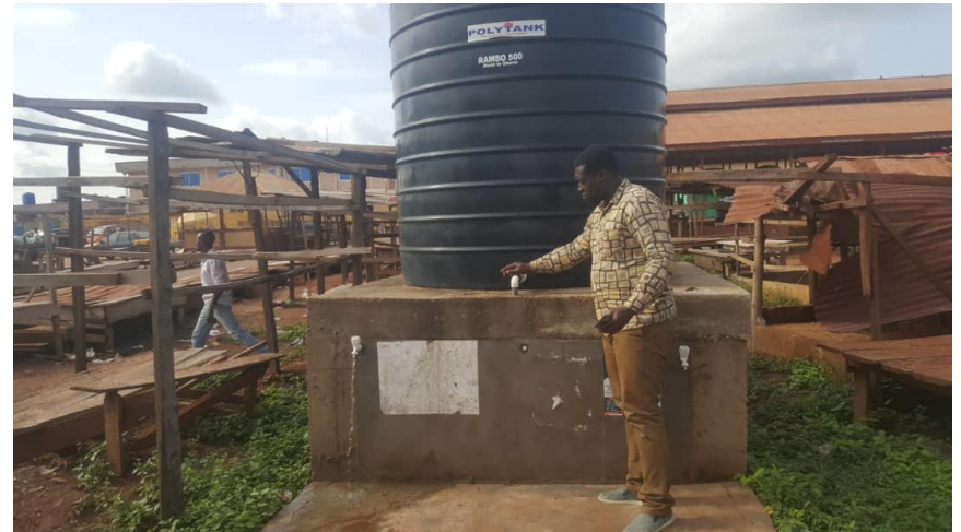
Figure 4: Borehole Mechanized at New Market (Wenchi)
