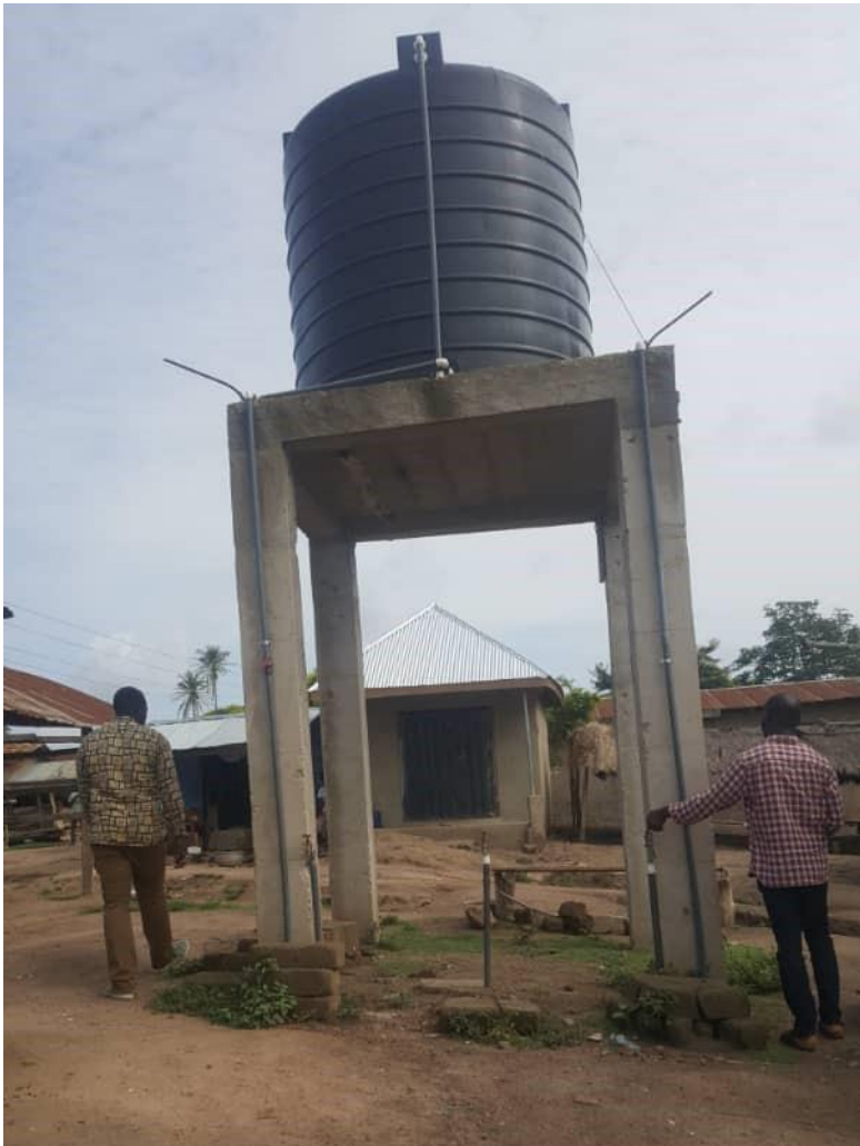
Figure 3: Mechanized Borehole constructed at Tromeso
