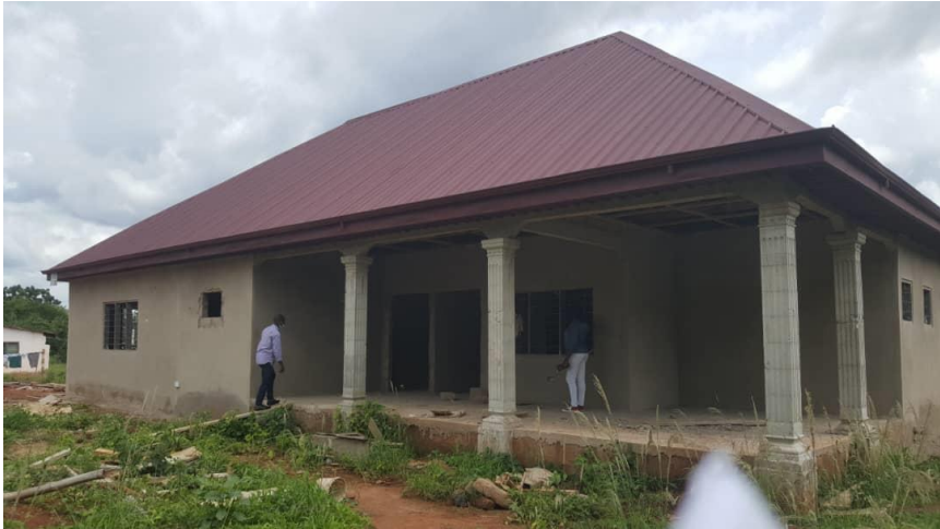
Figure 8: Construction and furnishing of 1 No Doctor's Quarters at Nchiraa
