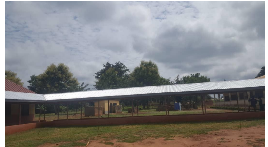
Figure 2: 65M Walkway constructed at Nchiraa Health Center
