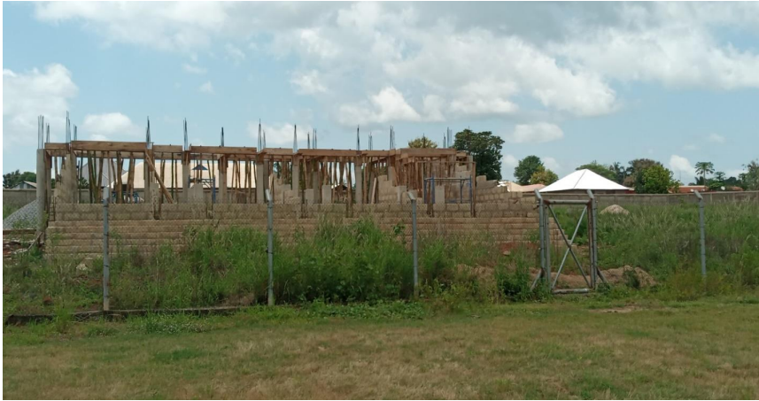
Figure 6: Construction of Spectators stands with press box at Wenchi Sports Field
