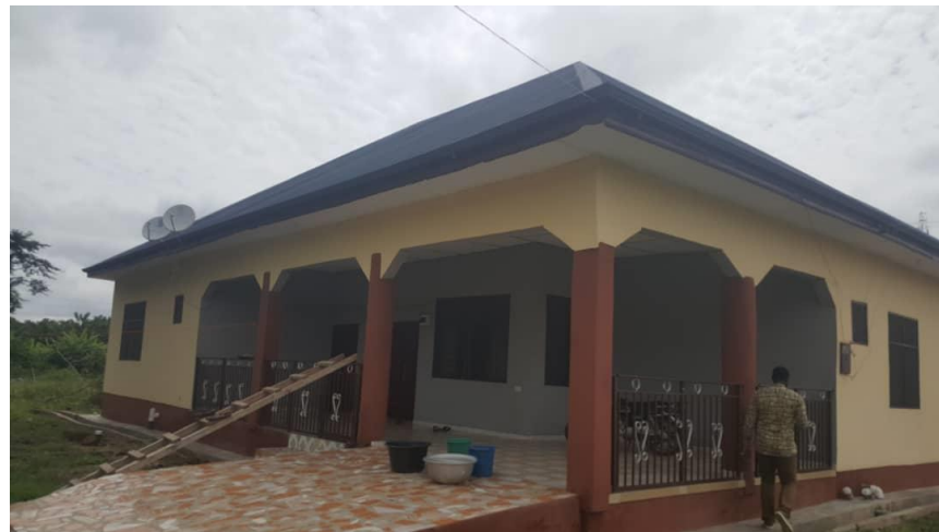
Figure 1: Doctor's quarters constructed at Subinso
