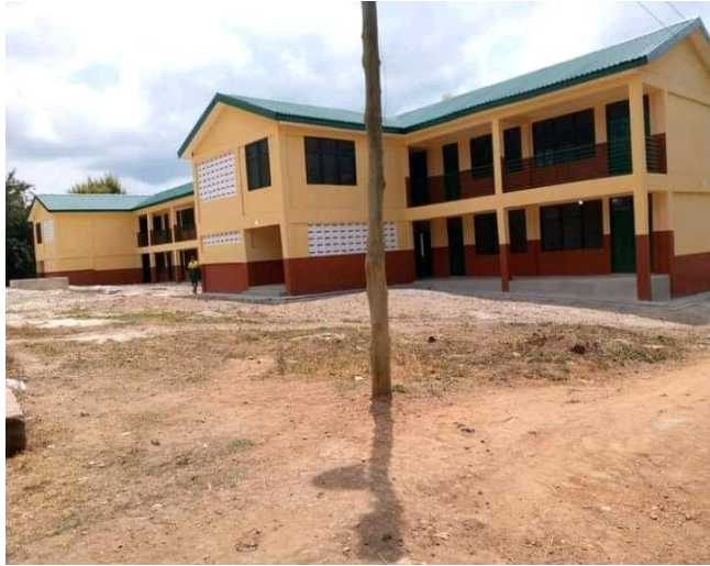
Project 8: Construction of 1 No. 3-unit classroom block at Ningokrom
