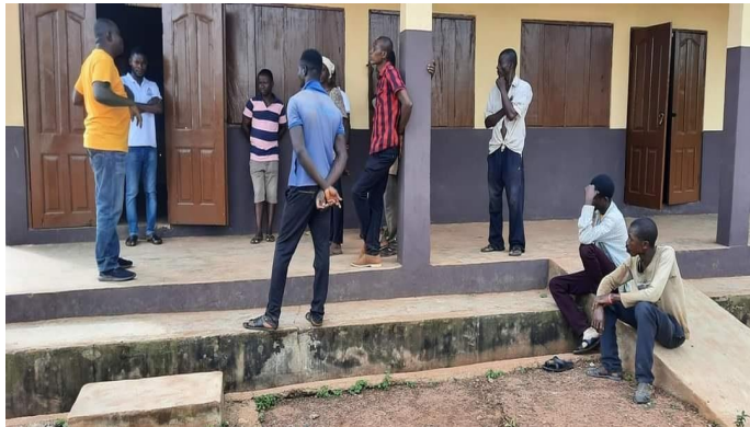
Project 9: Construction of 1 No. 3-unit KG block at Wamfie
