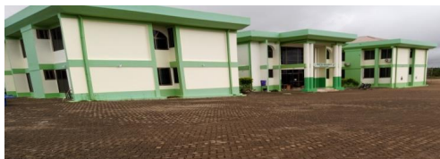
18. Renovated the Administration Block Complex and Guest House with Others of the Prestea Huni-Valley Municipal Assembly
