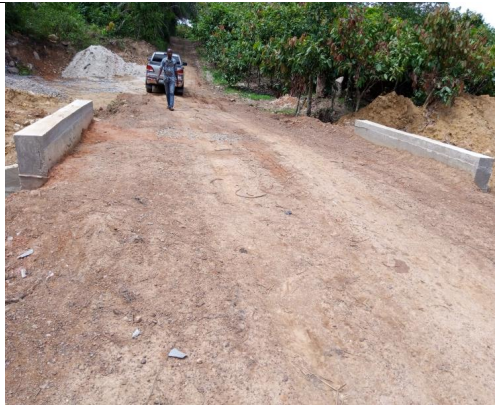
11. Constructed Double Cell Box Culvert on Baakoyemobo Road
