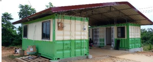
17. Creation of additional offices using Prefabricated Metal Containers for The Prestea Huni-Valley Municipal Assembly
