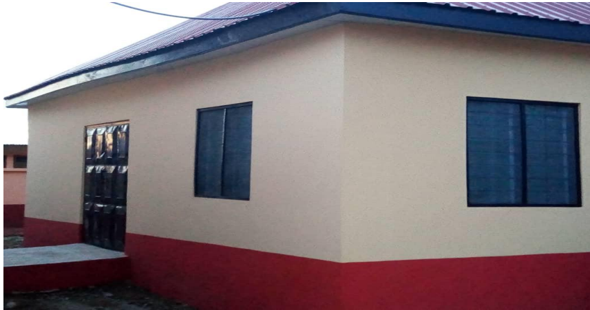
Figure 3: Construction of maternity ward at RCH
