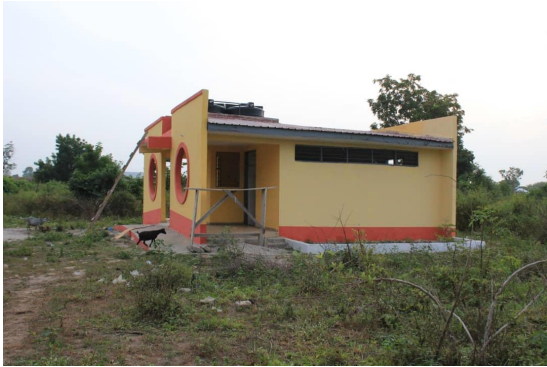
CONSTRUCTION OF TOILET AT BRODI-SPECIAL INITIATIVE
