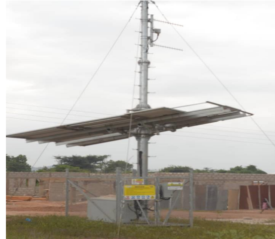
TELEPHONE MAST INSTALLED AT NAMASA-GIFEC
