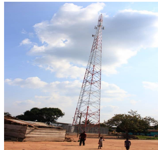
TELEPHONE MAST INSTALLED AT TANOKROM-GIFEC
