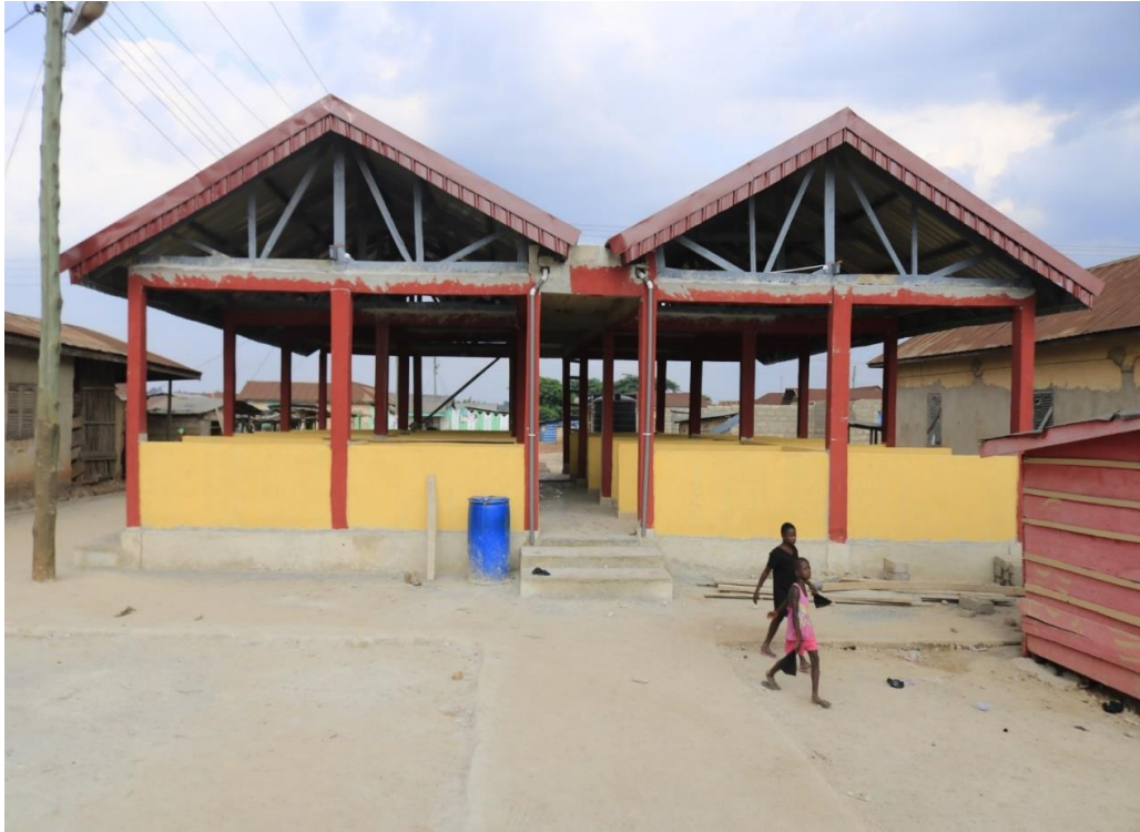
2NO.24 MARKET SHED CONSTRUCTED AT DORMAA AKWAMU AND AKONTANIM
