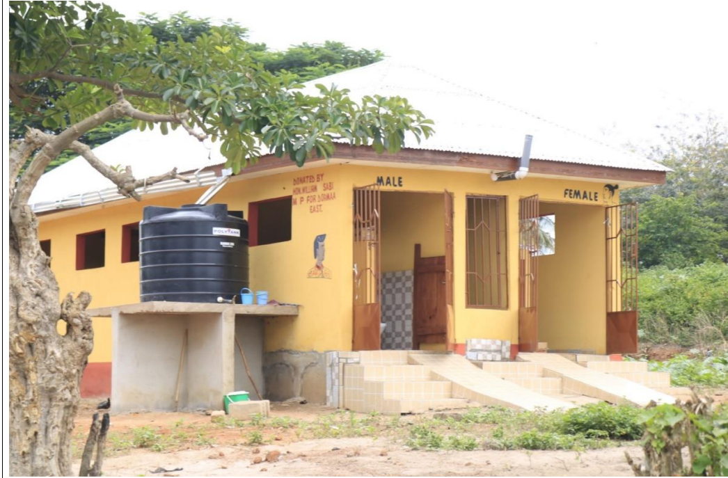
1NO 20-SEATER WATER CLOSET CONSTRUCTED
