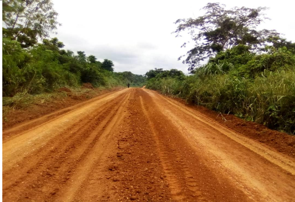
117 KM FEEDER ROAD RESHAPED
