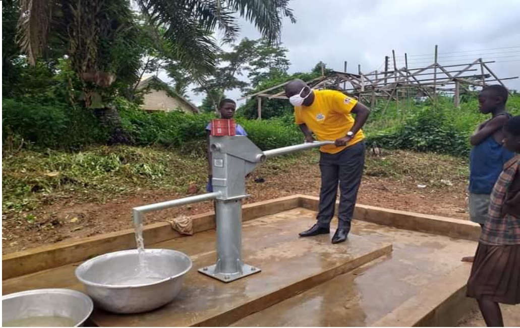
PROVISION OF PORTABLE WATER-COVID 19 INTERVENTION
