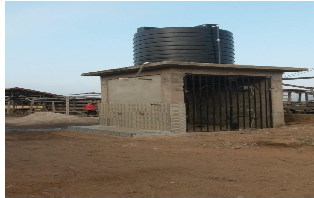
PROVISION OF WATER SYSTEM TO 6NO. MARKETS IN THE DISTRICT-COVID 19 INTERVENTION
