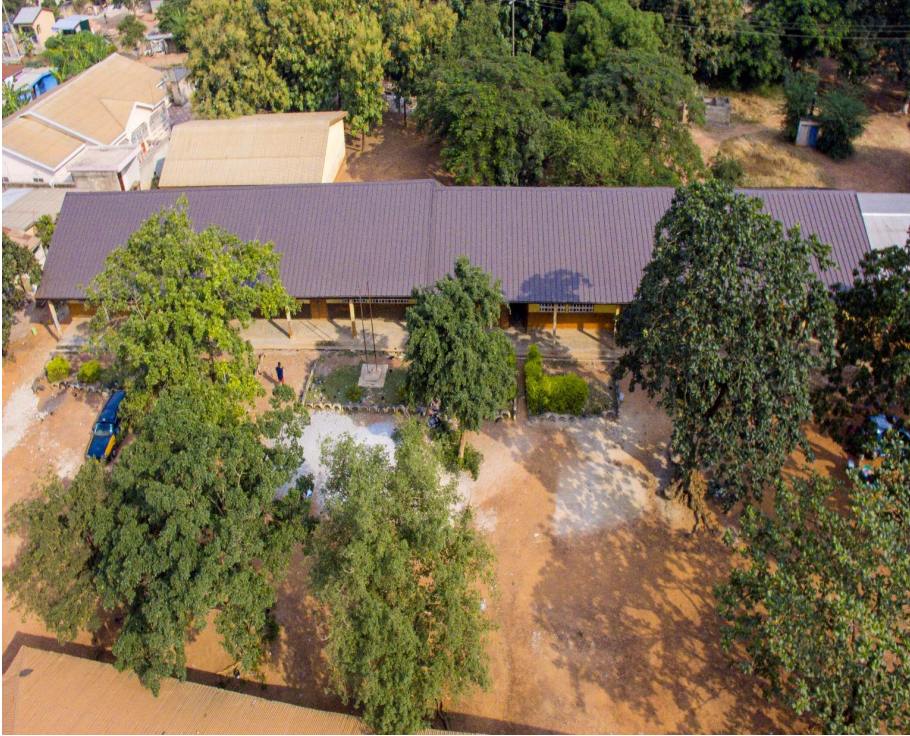
1no. Six Classroom Block at Nyankyerenease Renovated
