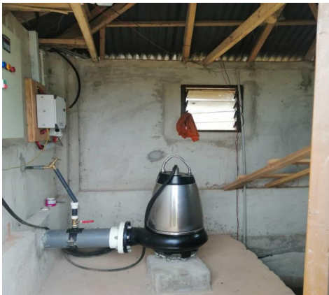
Figure 10: Installed Pump to Transfer Faecal Sludge
