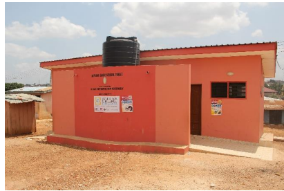
Figure 9. 10-seater institutional toilet at Anyaano Basic School
