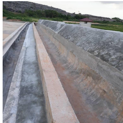
Figure 11: Additional Works On the Headworks for Faecal Sludge Discharge
