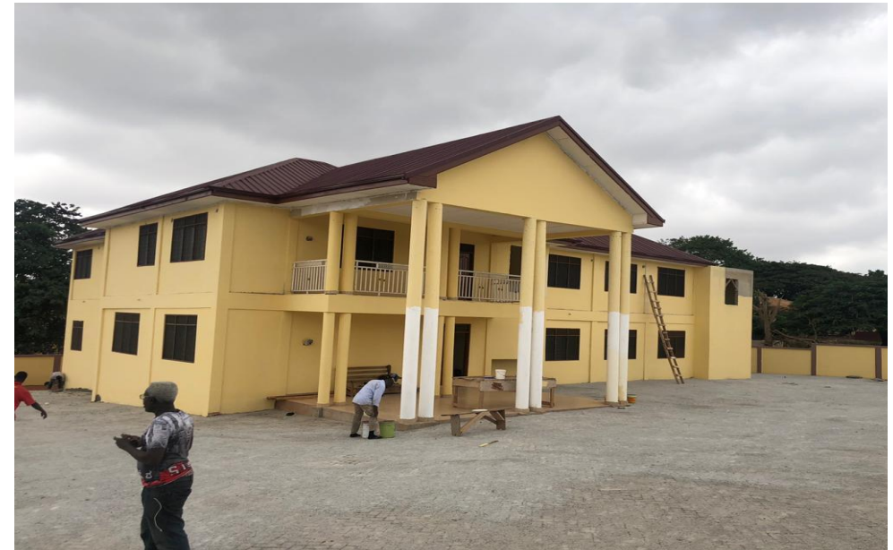
Figure 13: Constructed Nhyiaeso Sub-Metro Office at Fankyenebra.
