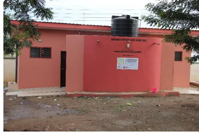
Figure 7. 10-seater institutional toilet at Bantama State Boys Basic School
