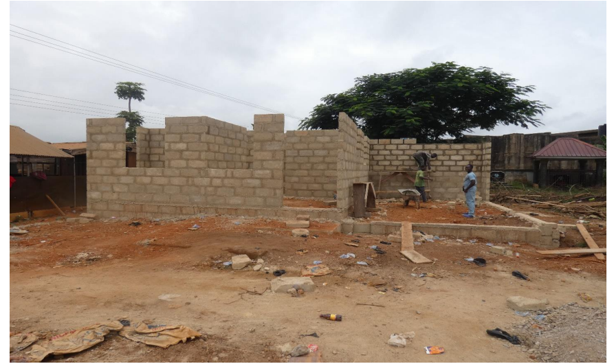
Construction of ambulance Bay at Bebu at lentil level.
