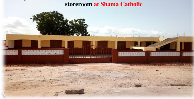
Completion of 3 unit Classroom Block with Head master's office and a storeroom at Shama Catholic
