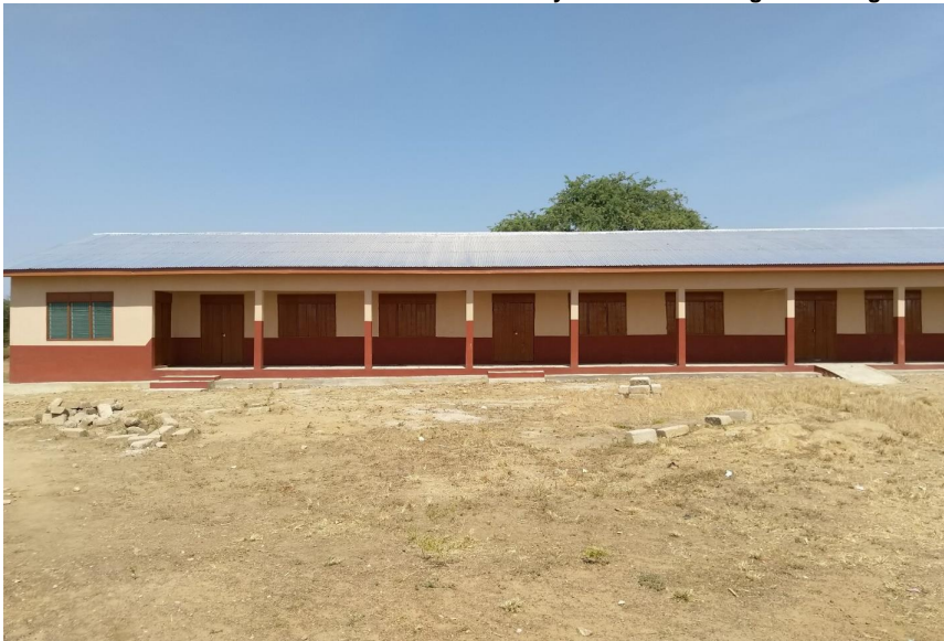
Construct1no. 3 - Unit classroom block with ancillary facilities at Sherigu Azaalunge
