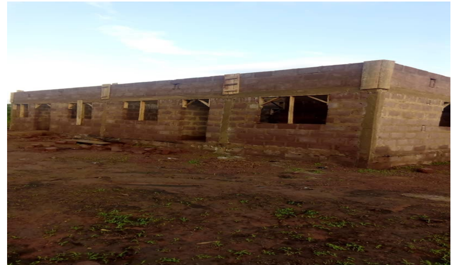
FIGURE 7: 2NO. CHPS COMPOUND CONSTRUCTED AT MANCHARE AND CEDIKOPE
