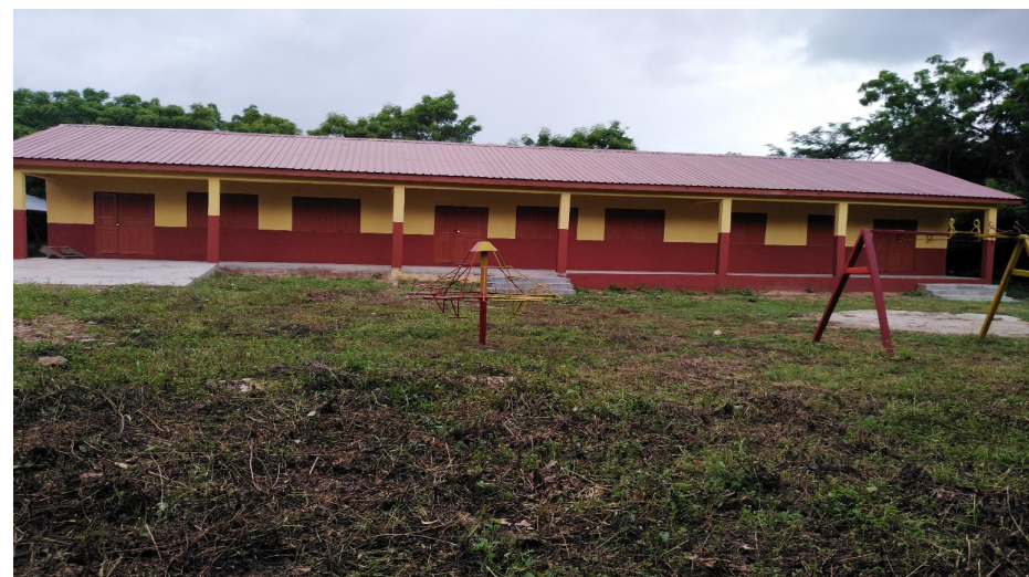
Figure 2: 2-UNIT KG BLOCK, OFFICE, STORE AND PLAY-GROUND CONSTRUCTED AT KAYERA
