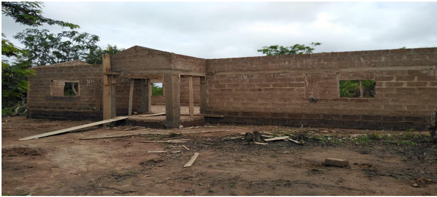
Figure 6: 1NO. SLAUGHTER HOUSE CONSTRUCTED AT ADEEMMRA
