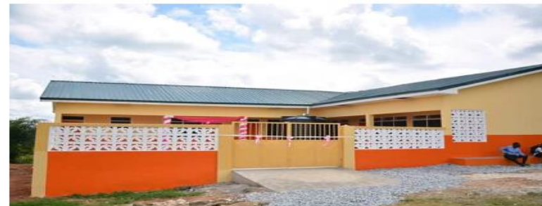
Newly Constructed Aboabo Salvation Army KG Block
