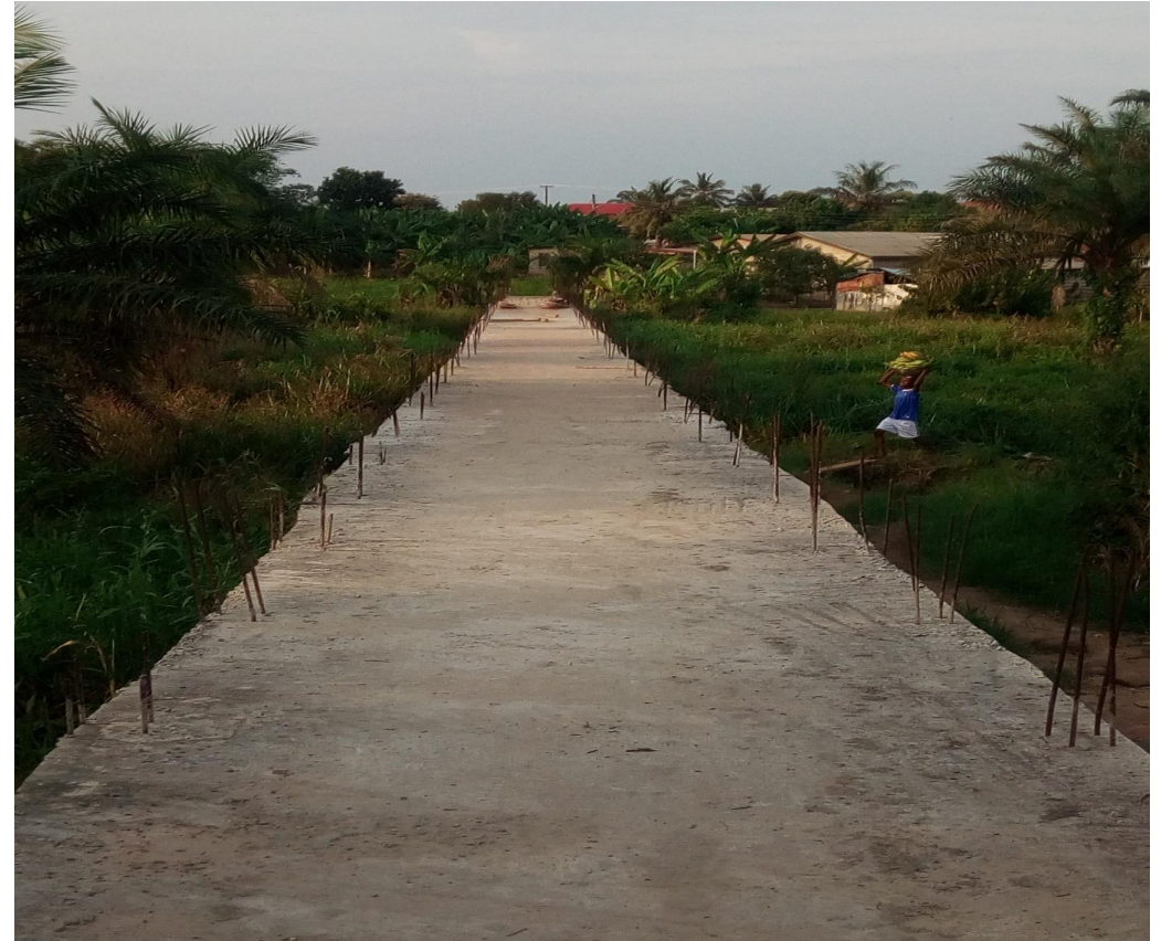
1 NO. FOOTBRIDGE UNDER CONSTRUCTION AT JESUS-JESUS, AKIM ODA
