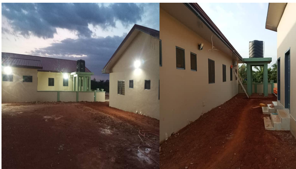
Completed CHPS Compound at Koforidua
