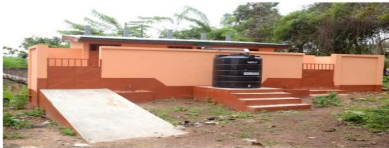
A toilet facility built by World Vision at Hwidiem
