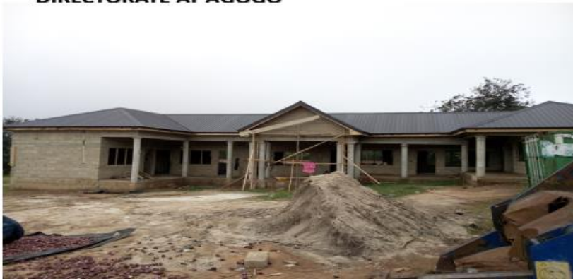
CONSTRUCTION OF DISTRICT HEALTH DIRECTORATE AT AGOGO
