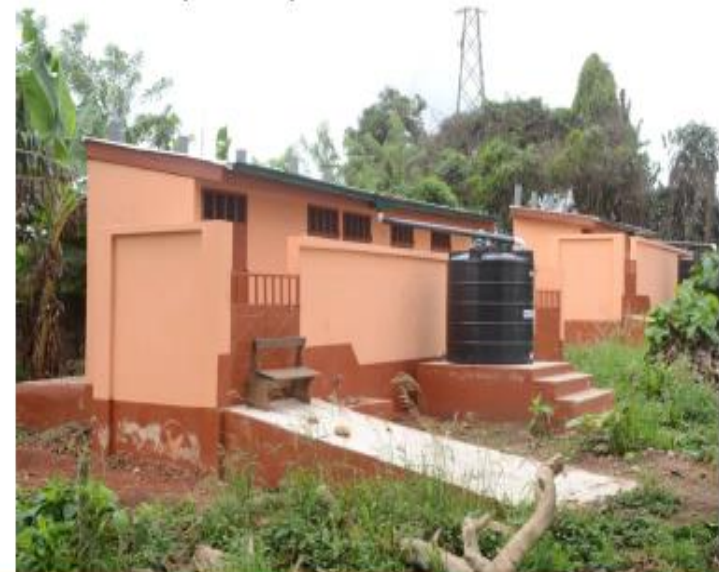
A toilet facility built by World Vision at Kowriso
