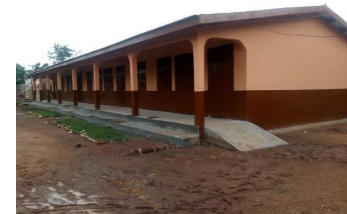
REHABILITATION OF 1NO. 6-UNIT CLASSROOM BLOCK WITH OFFICE, STORE, STAFF COMMONROOM AND LIBRARY AT ASUADEI
