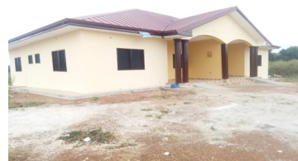
FACILITIES AT ADUGYAMA
