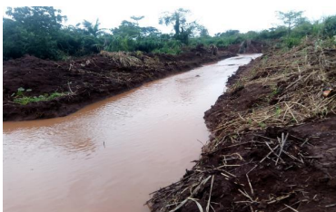
DREDGING OF ESURENFUOR RIVER AT SABRONUM
