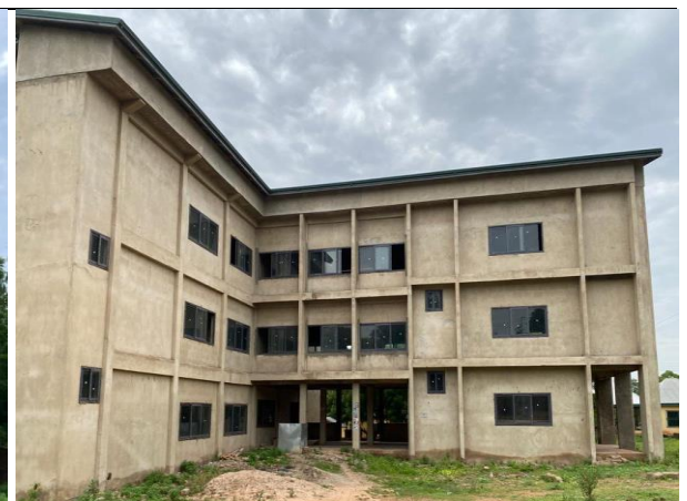
Figure 3: Progress on the Tamale Regional Office Project
