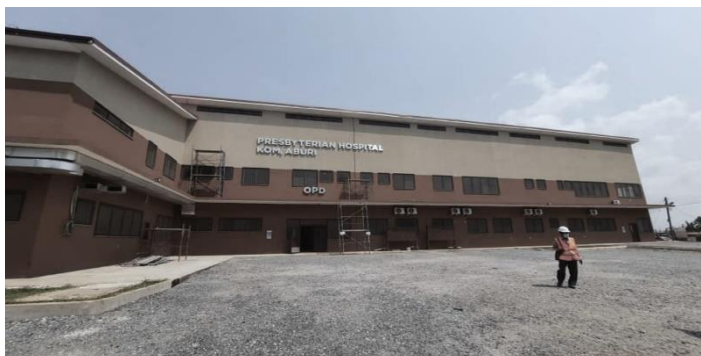
Modernisation and Equipping of Aburi Hospital
