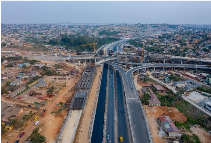
Pokuase Interchange (Accra Urban Transport Project)
